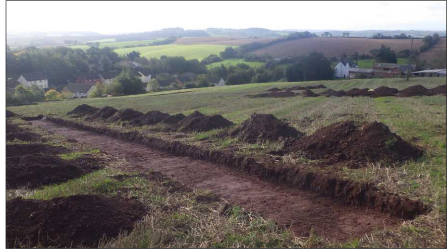
Plate 2: General view of site in the vicinity of Trench 14, looking southwest
