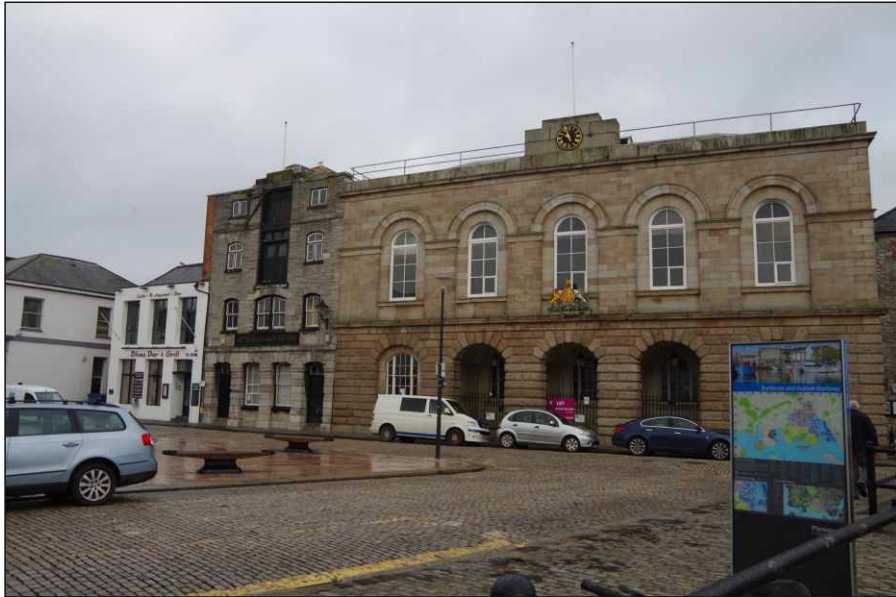
Plate 1: General view of the building showing the Custom House to the east, looking northwest (1m scale)
