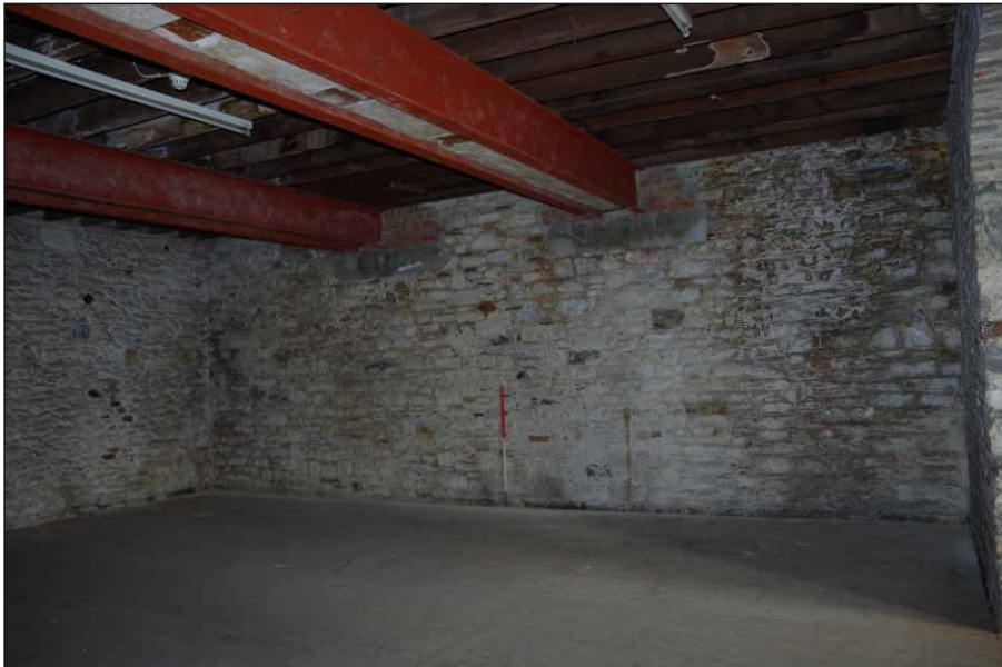
Plate 14: Second-floor east wall of central store, looking northeast (1m scale)
