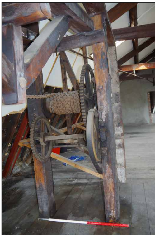
Plate 16: Cogs and chains of winch arm in the third-floor south store, looking northwest (1m scale)
