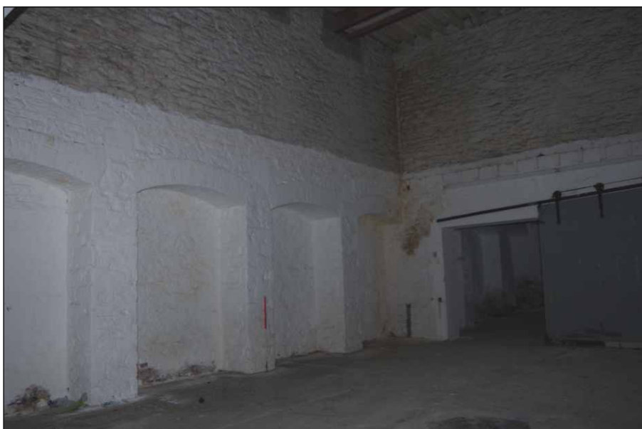
Plate 9: Ground-floor east wall of north store, looking southeast (1m scale)
