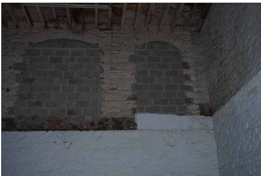
Plate 8: First-floor south wall of south store, looking south
