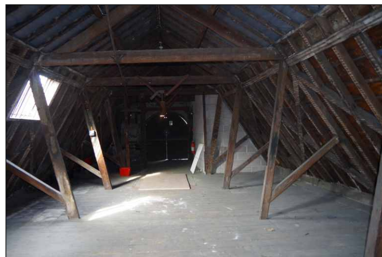
Plate 19: General view of roof structure, looking north
