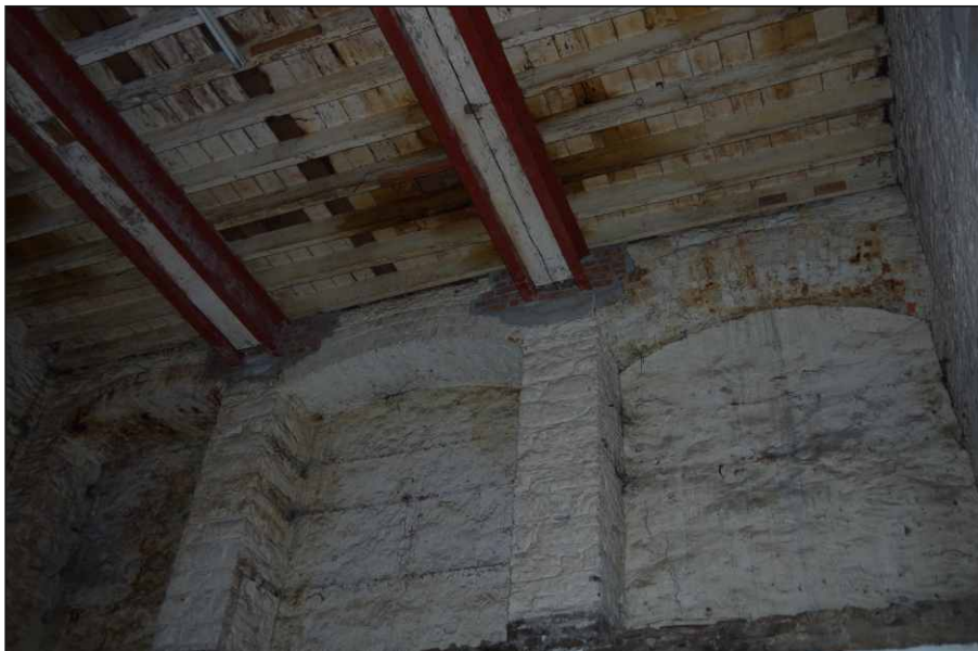
Plate 7: First-floor east wall of the south store, looking northeast
