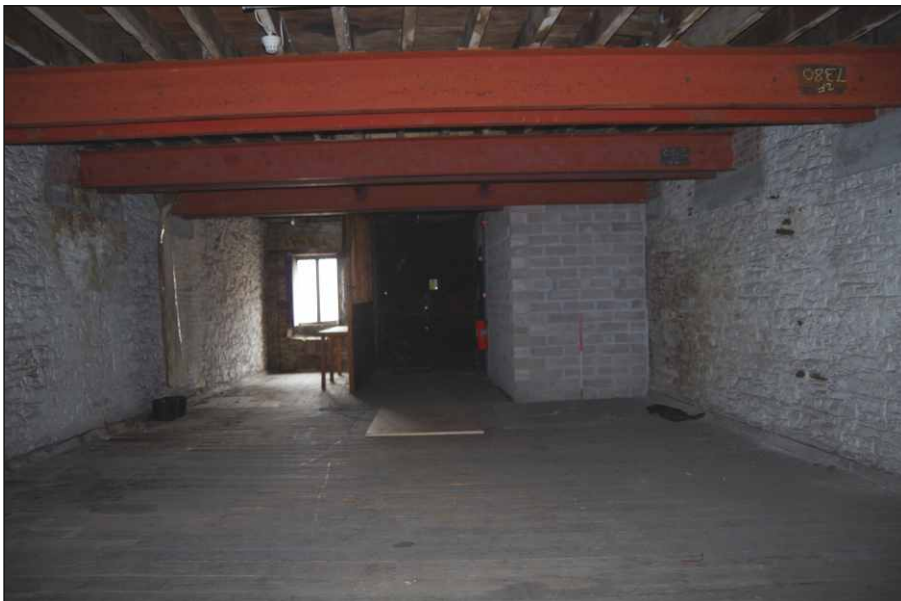
Plate 15: General view of second-floor north store, looking north (1m scale)
