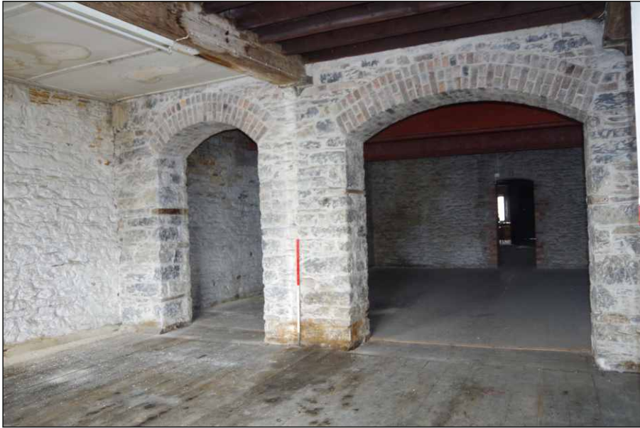
Plate 13: Second-floor north wall of the south store, looking northwest (1m scale)
