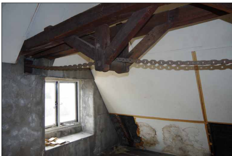
Plate 17: Chain of winch arm in the third-floor south store, looking southwest
