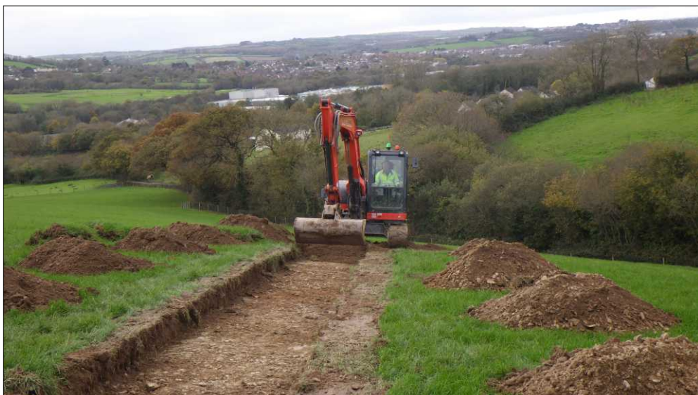
Plate 3: Showing working view of Trench 1, looking southwest
