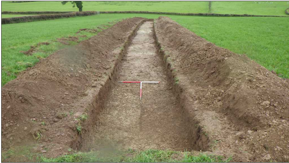
Plate 4: Trench 2, view to southwest (scales 1m)
