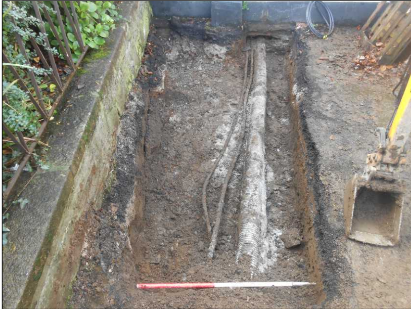
Plate 3: The excavated joint pit, looking southeast. 1m scale
