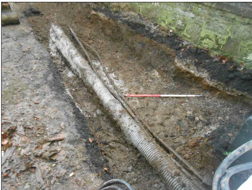
Plate 4: The excavated joint pit, looking east. 1m scale
