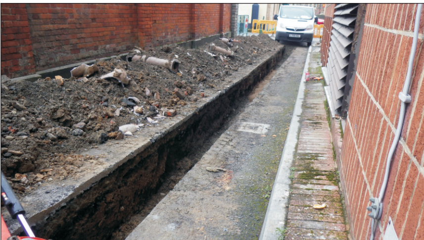
Plate 3: Showing cable trench. View to south
