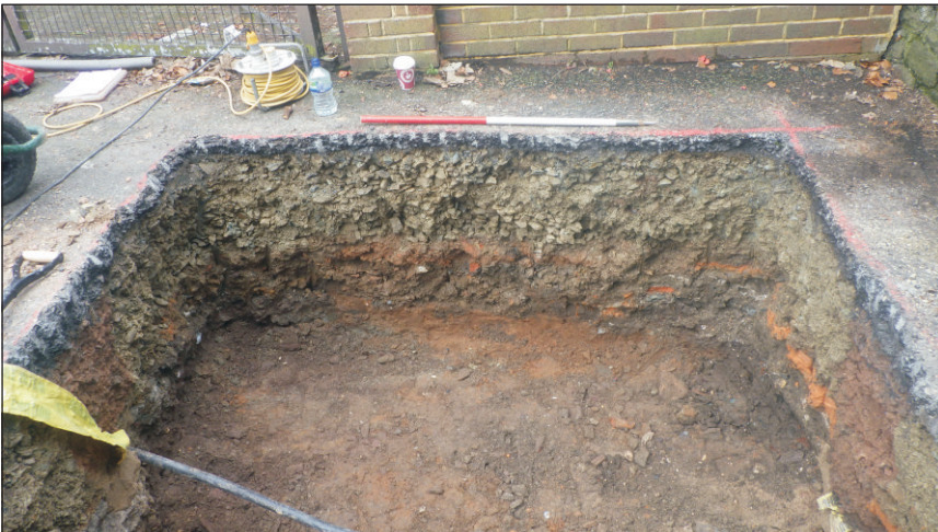
Plate 2: Showing substation trench. View to west (scale 1m)
