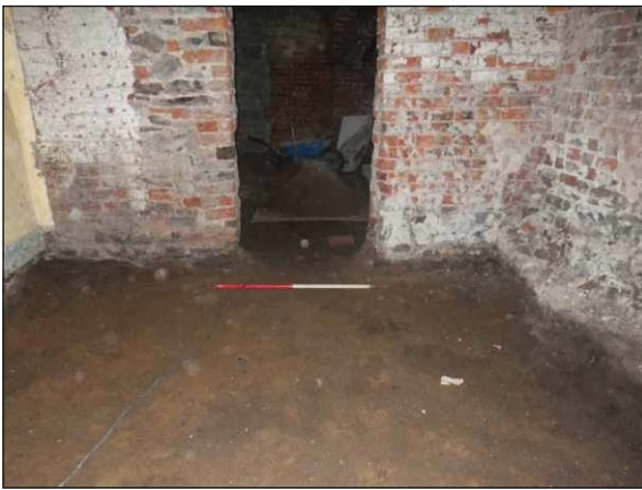
Plate 2: Room 1, view to west following floor reduction (scale 1m)
