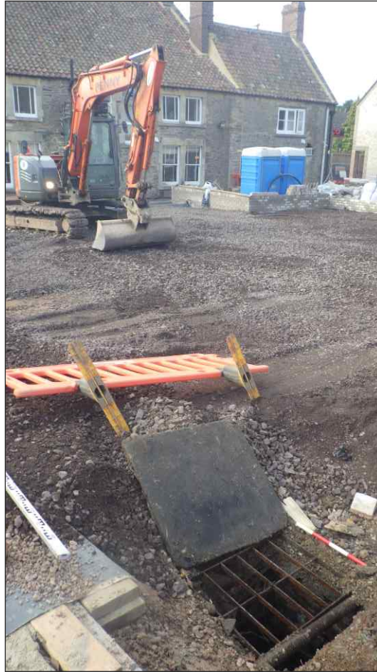
Plate 6: Manhole for access to subterranean tank, looking west (0.4m scale)
