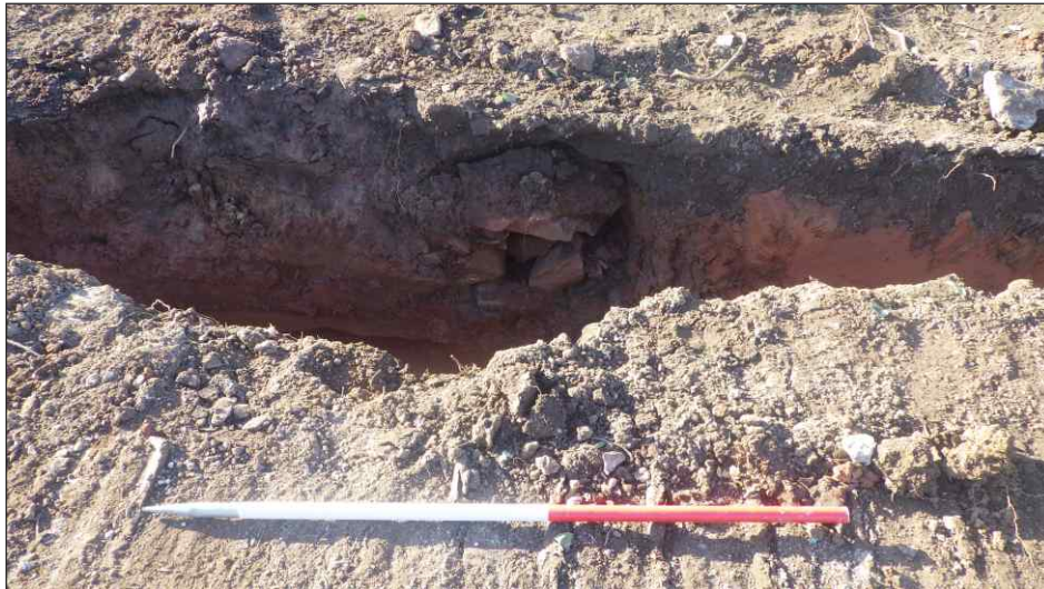
Plate 4: Northeast-facing section of land drain in northeast part of the site (1m scale)
