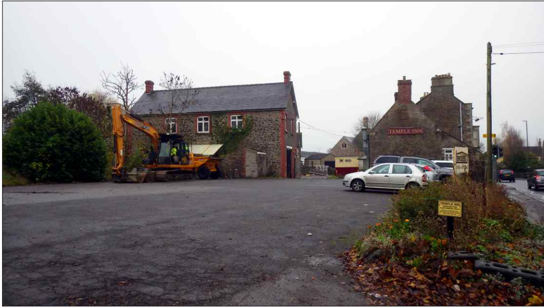
Plate 1: General site view, looking southeast
