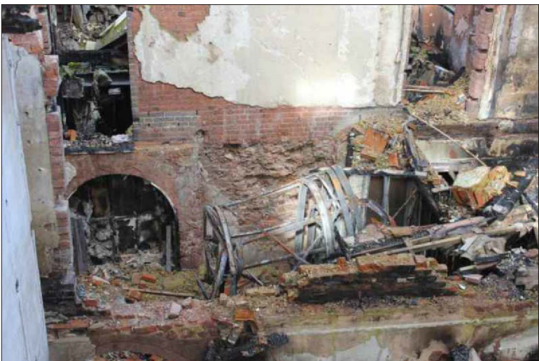
Plate 29: The central area of the ground floor, looking northeast
