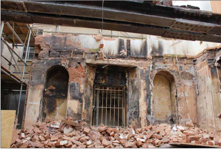
Plate 36: The ground floor, north range, northwest wall, looking northwest
