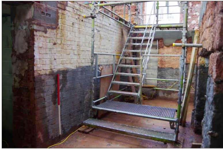
Plate 16: The front basement, looking northwest. (1m scale)
