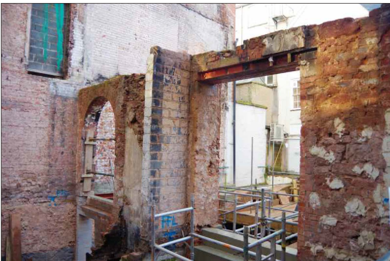
Plate 32: The ground-floor middle range, northwest wall, looking west
