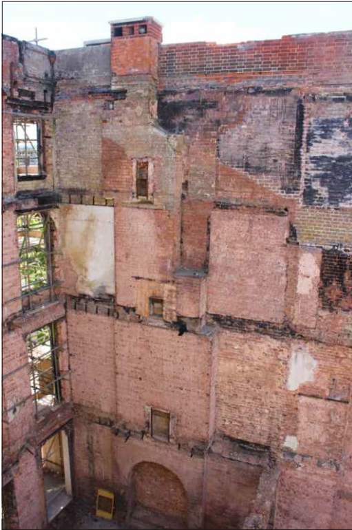
Plate 45: The southwest elevation of the north range, looking south
