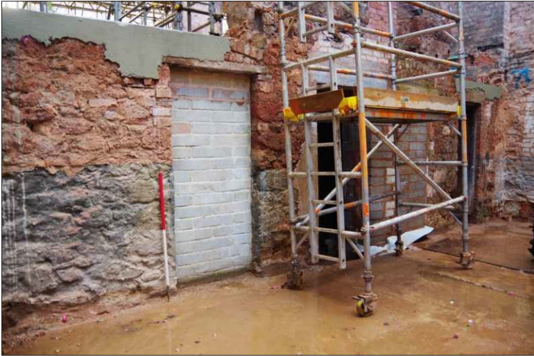
Plate 7: The middle basement, southeast wall, looking south. (1m scale)
