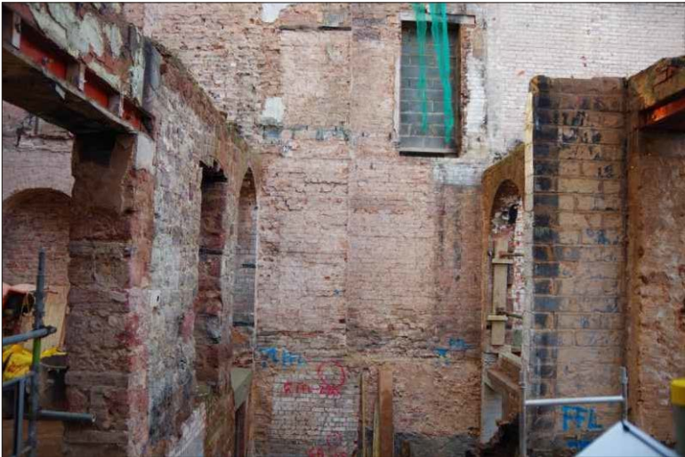
Plate 31: The ground-floor middle range, southwest wall, looking southwest
