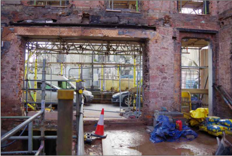
Plate 24: The ground-floor front range, southeast wall, looking southeast
