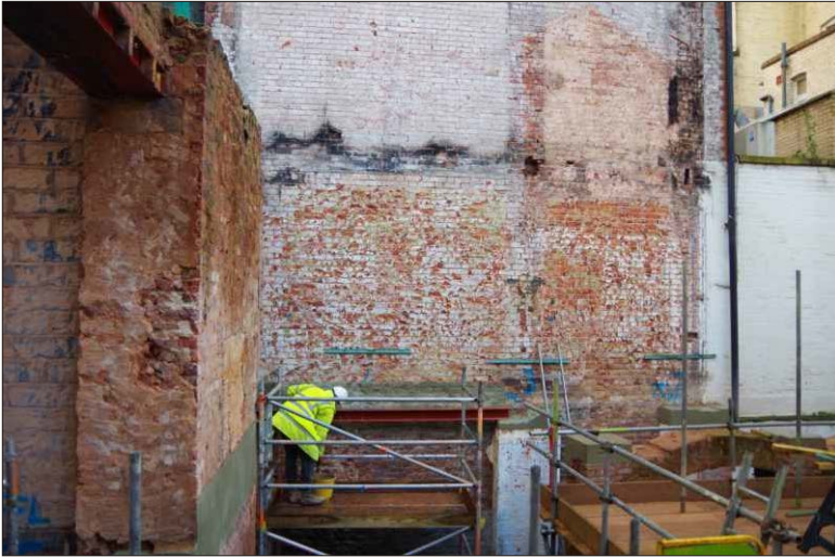
Plate 33: The ground floor, north range, southwest wall, looking southwest
