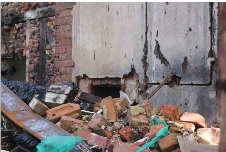
Plate 38: The first-floor front room southeast fireplace, looking east-northeast
