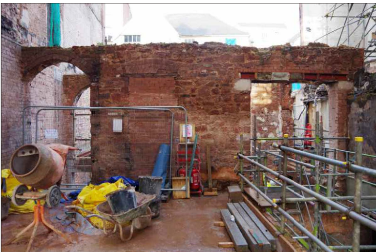
Plate 26: The ground-floor front range, northwest wall, looking northwest
