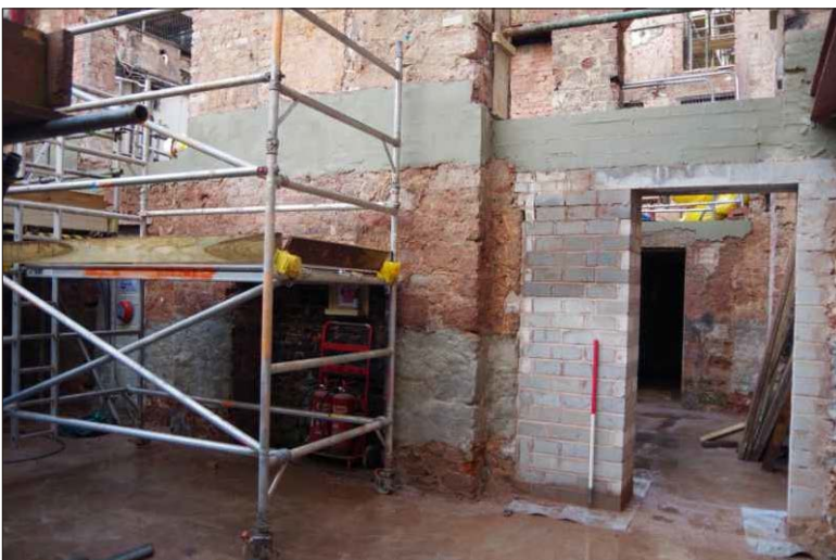
Plate 3: The rear basement, southeast wall showing fireplace, looking east. (1m scale)
