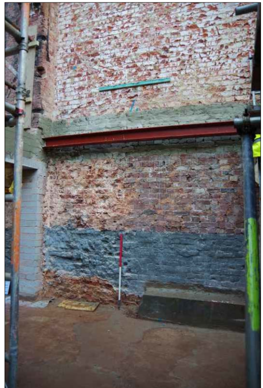
Plate 6: The rear basement, southwest wall, looking southwest. (1m scale)
