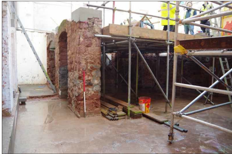
Plate 4: The rear basement showing the arched-headed piers, looking north. (1m scale)
