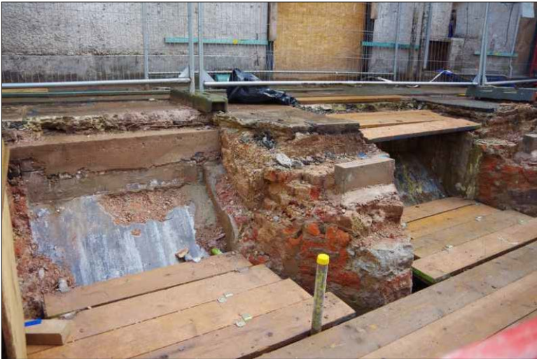
Plate 37: The ground floor, north range, base of northeast wall, looking east
