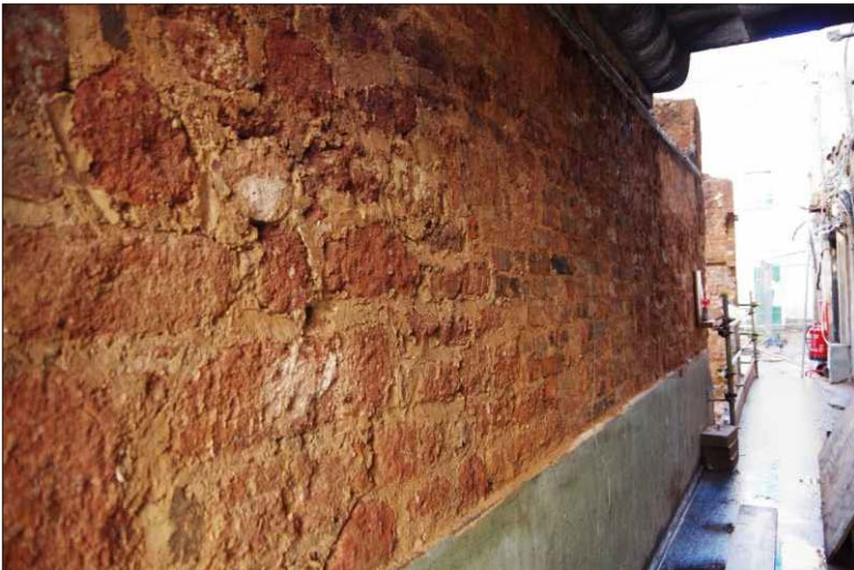
Plate 28: The ground-floor Lamb Alley passage showing brickwork in the rear of the front range fireplace, looking west
