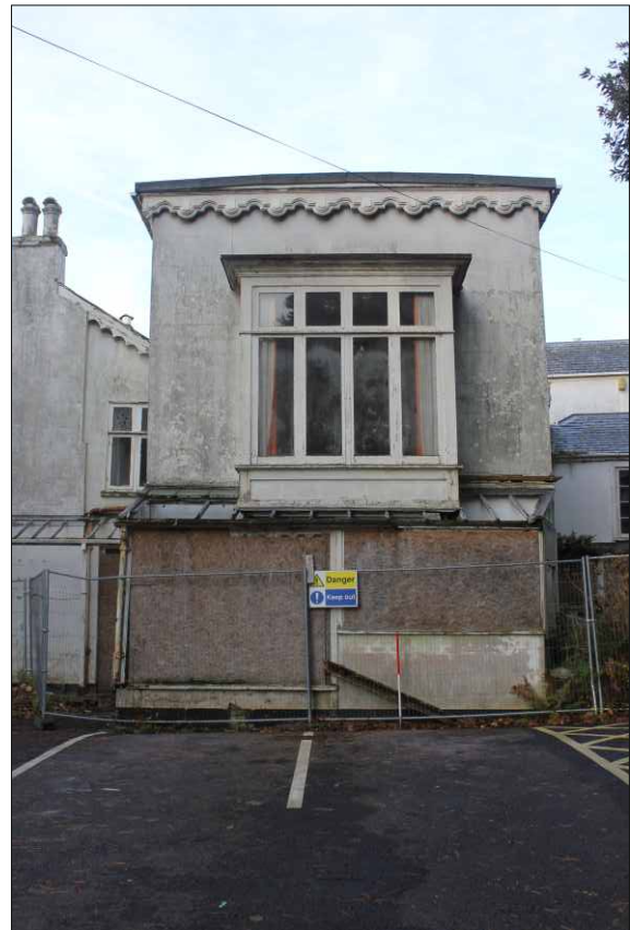
Plate 12: The east elevation of the house, looking west (1m scale)
