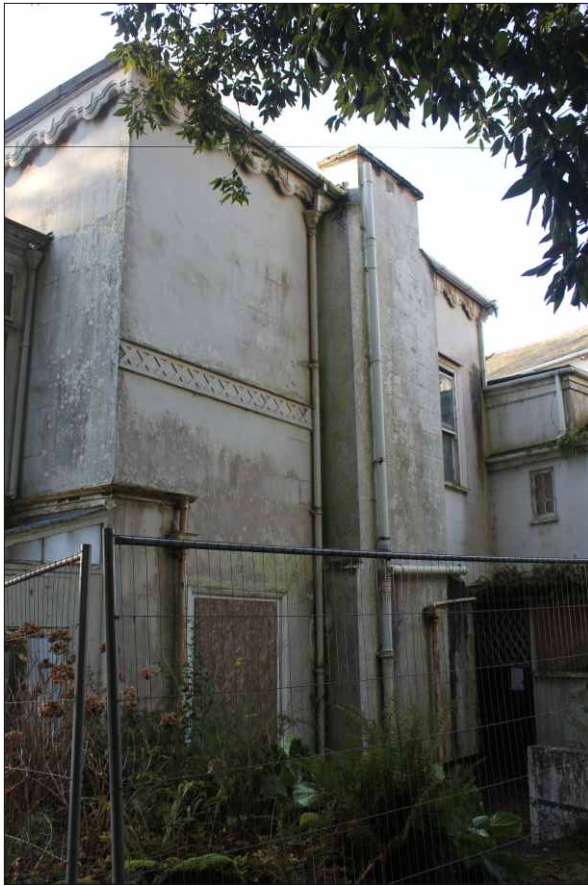
Plate 13: The north elevation of the main house, looking southwest
