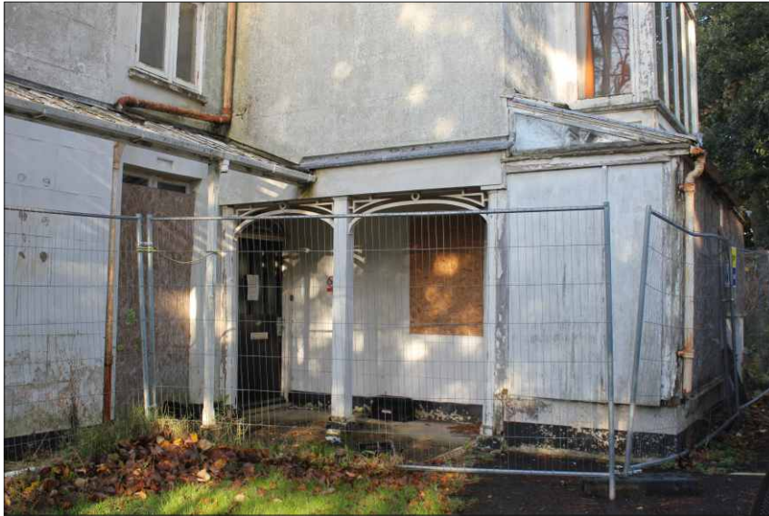
Plate 10: The entrance porch, looking northwest
