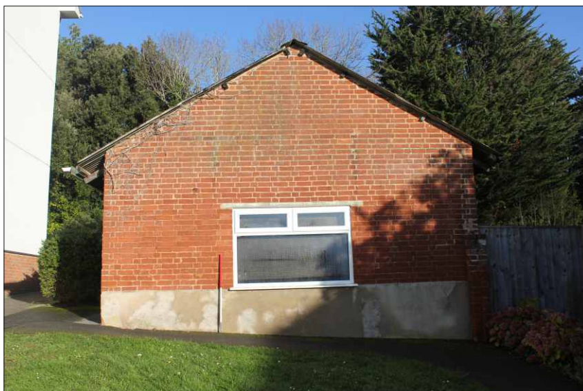
Plate 18: The south elevation of the stable block, looking north (1m scale)
