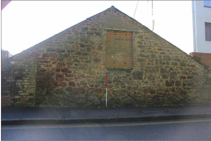
Plate 19: The north elevation of the stable block, looking south (1m scale)
