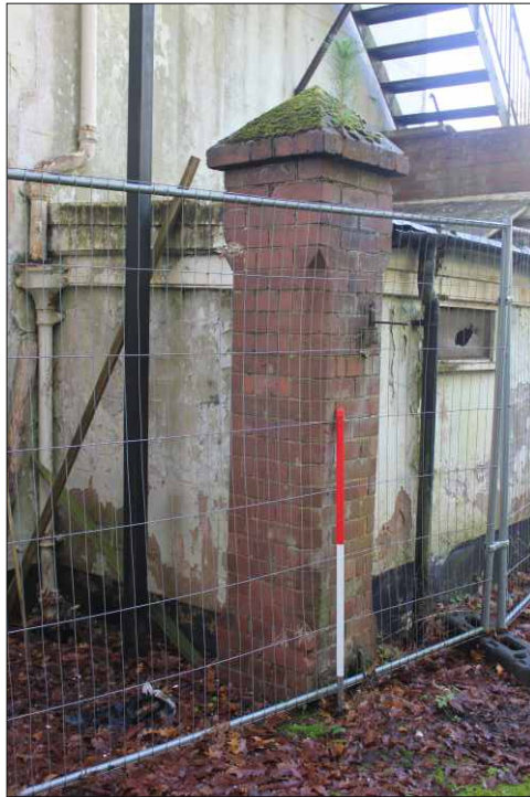
Plate 16: The gate pier incorporated into the rear extension, looking southwest (1m scale)
