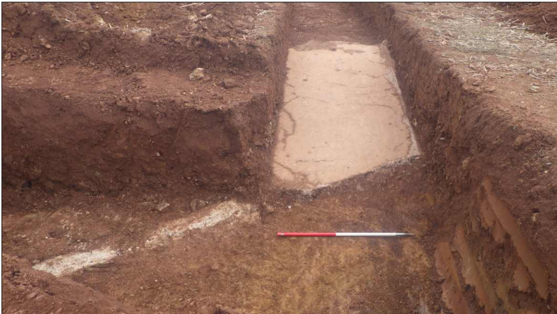
Plate 4: Trench 12, Structure 1, showing wall footing 1207 and floor surface 1205, looking southeast (scale 1m)
