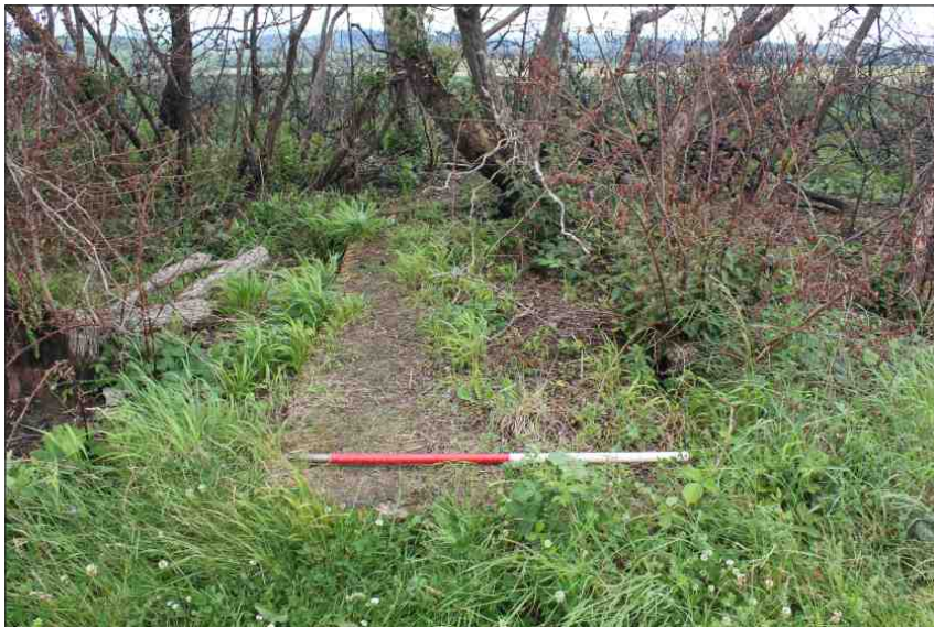
Plate 2: MDV70404, concrete base, looking southeast (1m scale)
