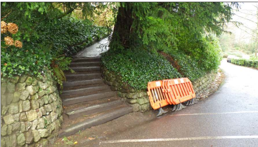
Plate 3: Pre-works view of Dunster Steps 2 (Upper Steps). View to northwest
