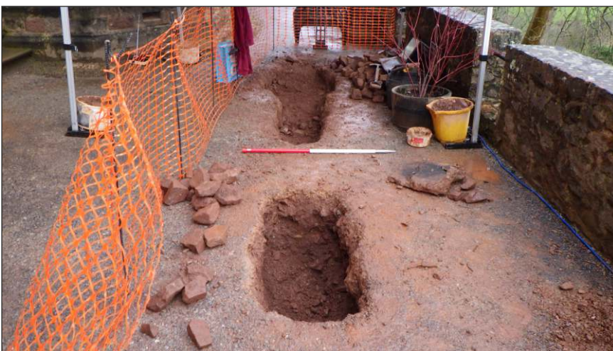
Plate 6: Showing pipe location test pits. View to northeast (scale 1m)
