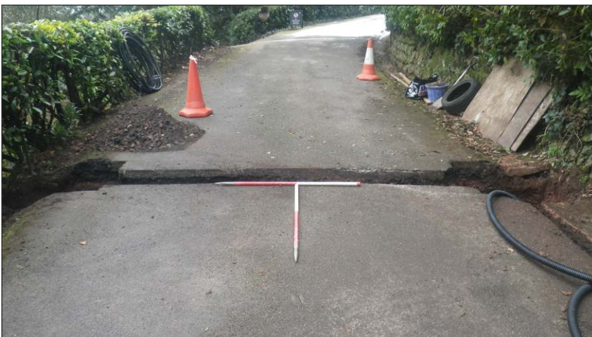
Plate 9: Electric gate installation works. View to south (scale 2x1m)
