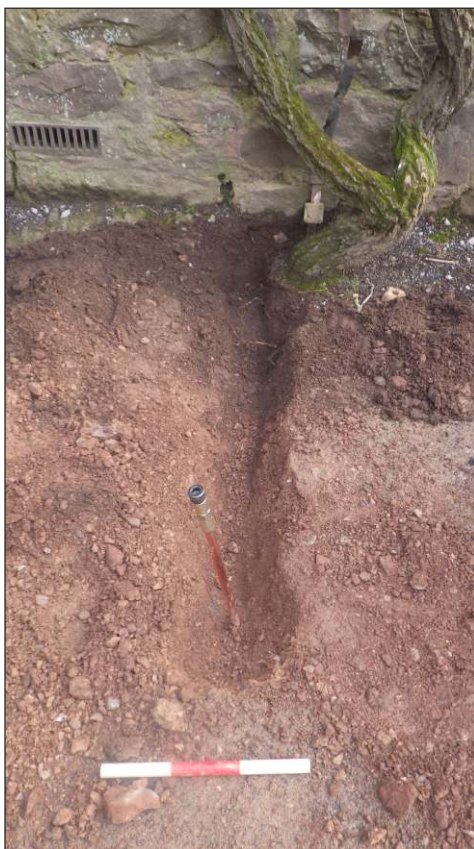
Plate 8: Lightning rod installation trench. View to northeast (scale 0.3m)
