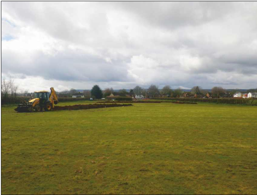
Plate 1: General view of the site, work in progress, looking southwest
