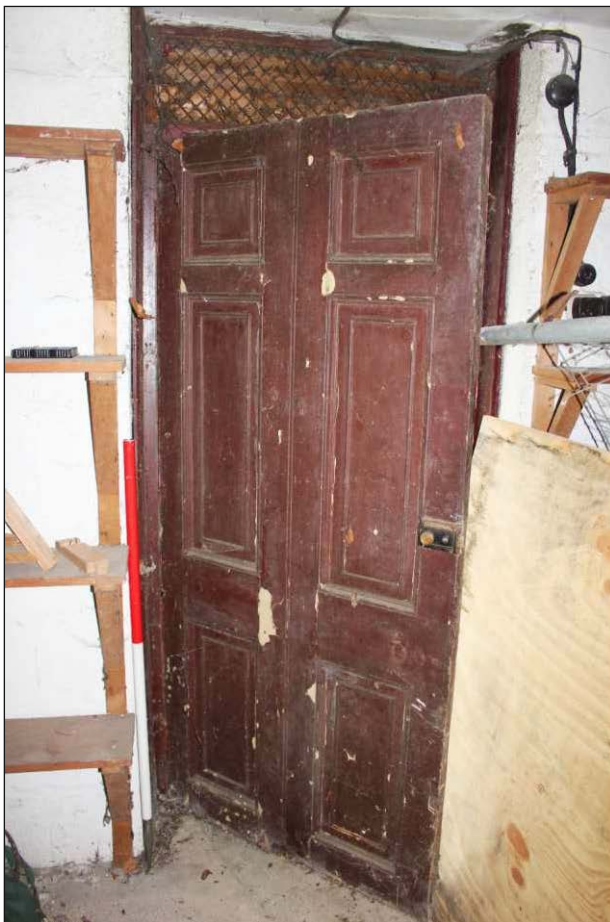
Plate 6: The reused six-panel door, looking east (1m scale)
