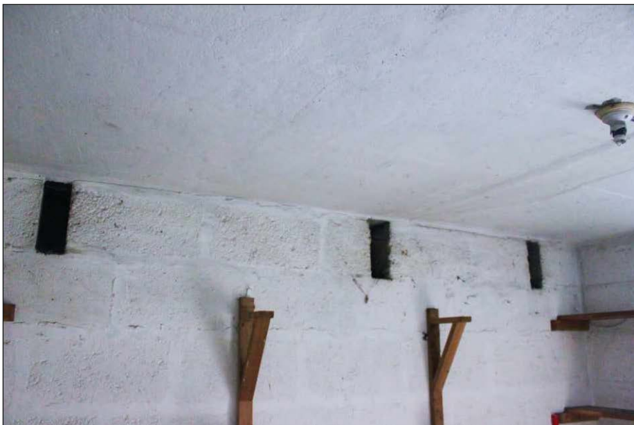
Plate 4: The northwest internal elevation showing vents, looking north
