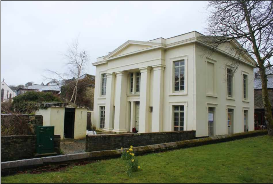
Plate 1: 1 Church Lane showing the outbuilding within the yard, looking northwest
