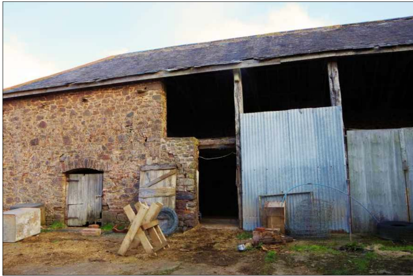
Plate 4: General view of south elevation of the north range, looking north
