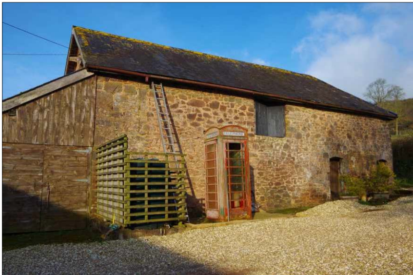
Plate 8: General view of east elevation of the east range, looking northwest
