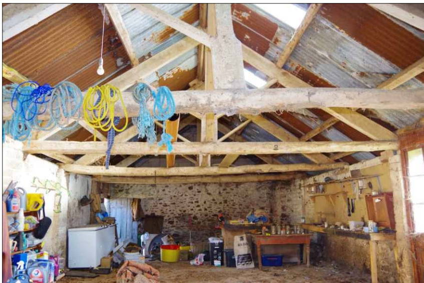
Plate 18: General view of the garage/store, looking east (1m scale)
