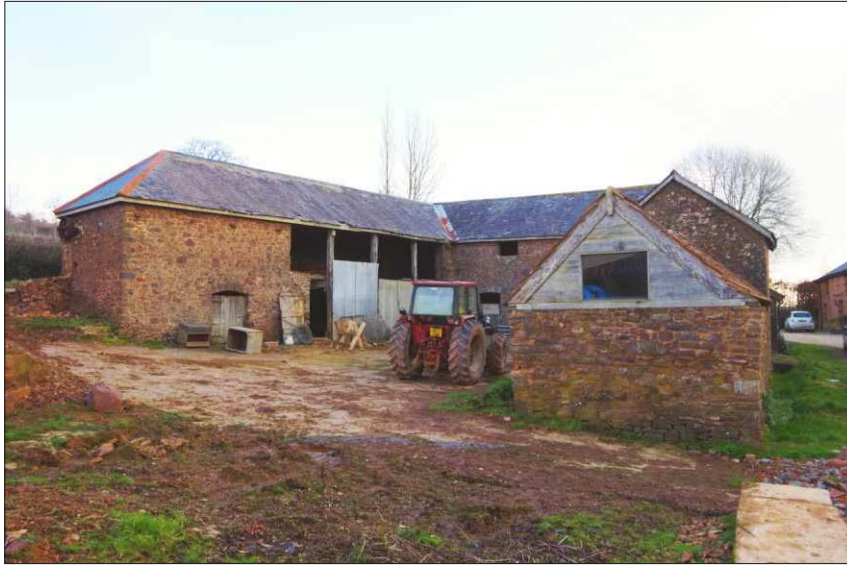
Plate 1: General view of barns, looking northeast
