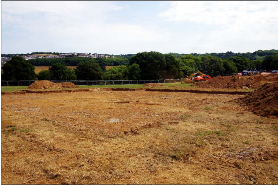
Plate 4: Excavation Area 1, looking southeast (1m scale)
