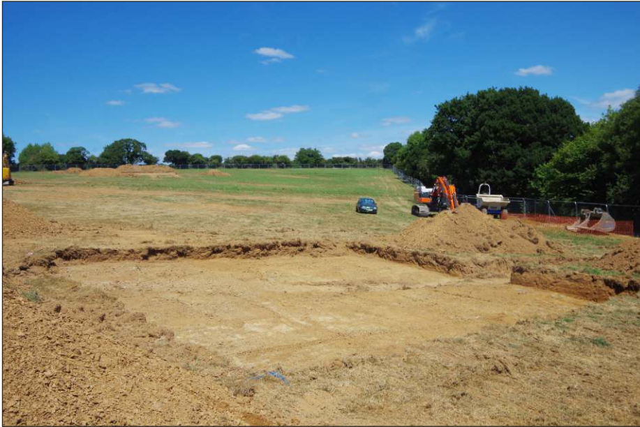
Plate 10: Excavation Area 2, looking northeast
