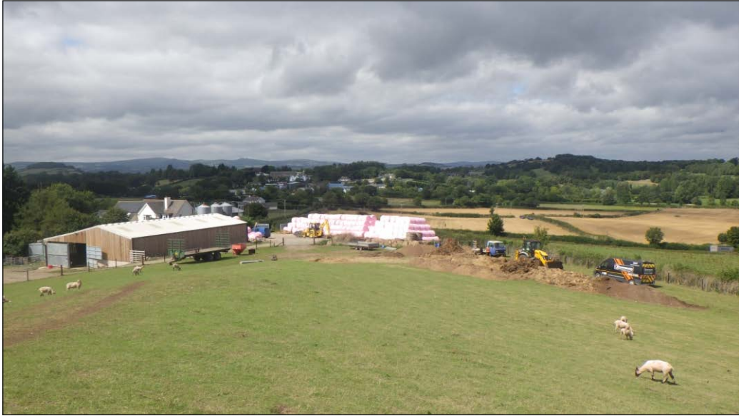
Plate 1: General working view of site. Looking northwest
