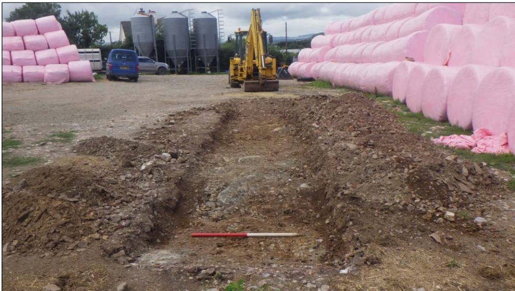
Plate 2: Trench 1, view to northwest (scale 1m)
