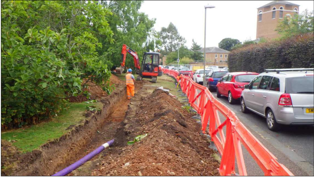
Plate 1: General working view of service trench excavations. Looking southeast
