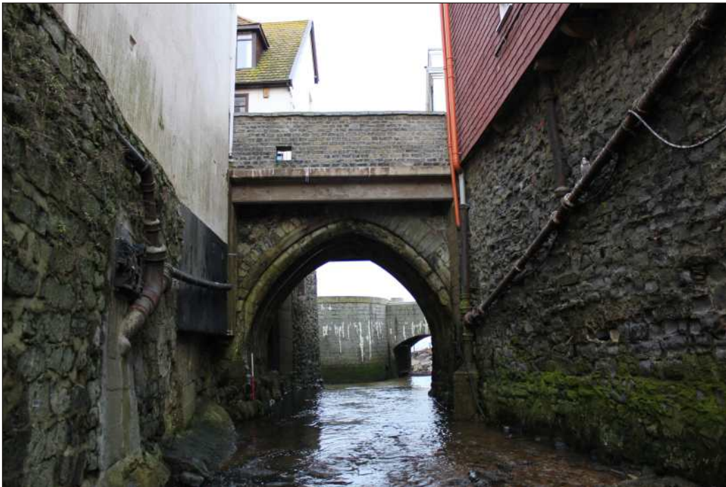
Plate 2: View of the bridge from the north (scale 1m)
