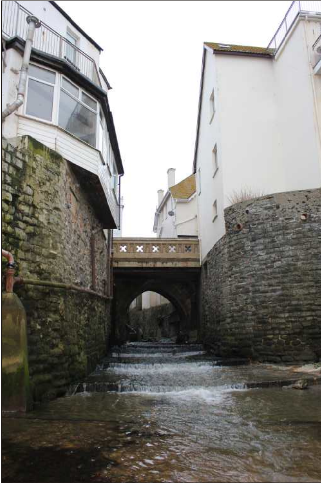
Plate 1: General view of the bridge from the south
