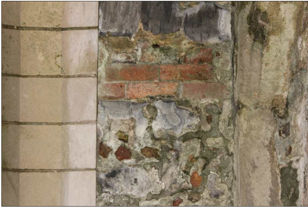
Plate 13: Repairs between ribs 3 and 4 on the west side of the bridge
