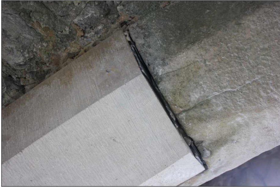
Appendix Plate 7: Rib 3 showing packing between stones, viewed from the northwest
