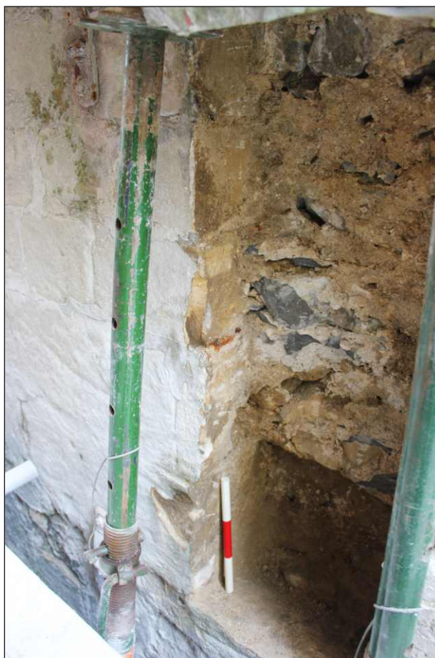
Appendix Plate 17: Rib 1 following removal of stones 1W:3 and 1W:4 and repair 125 showing masonry 100, viewed from the north. (0.30m scale)
