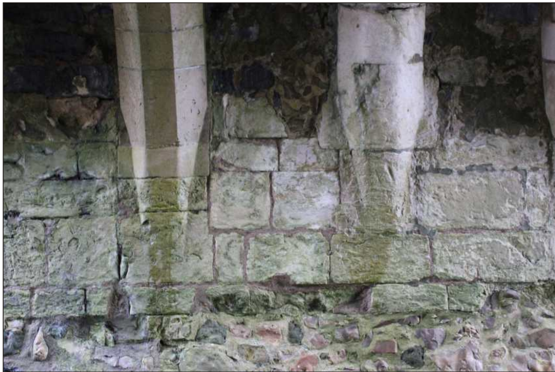
Plate 3: East side squared blocks between ribs 2 and 3
