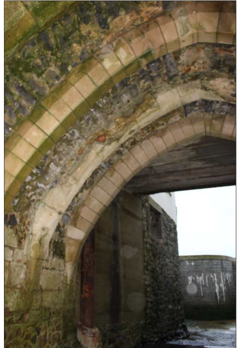
Plate 20: The northern face of the east side of Rib 3
