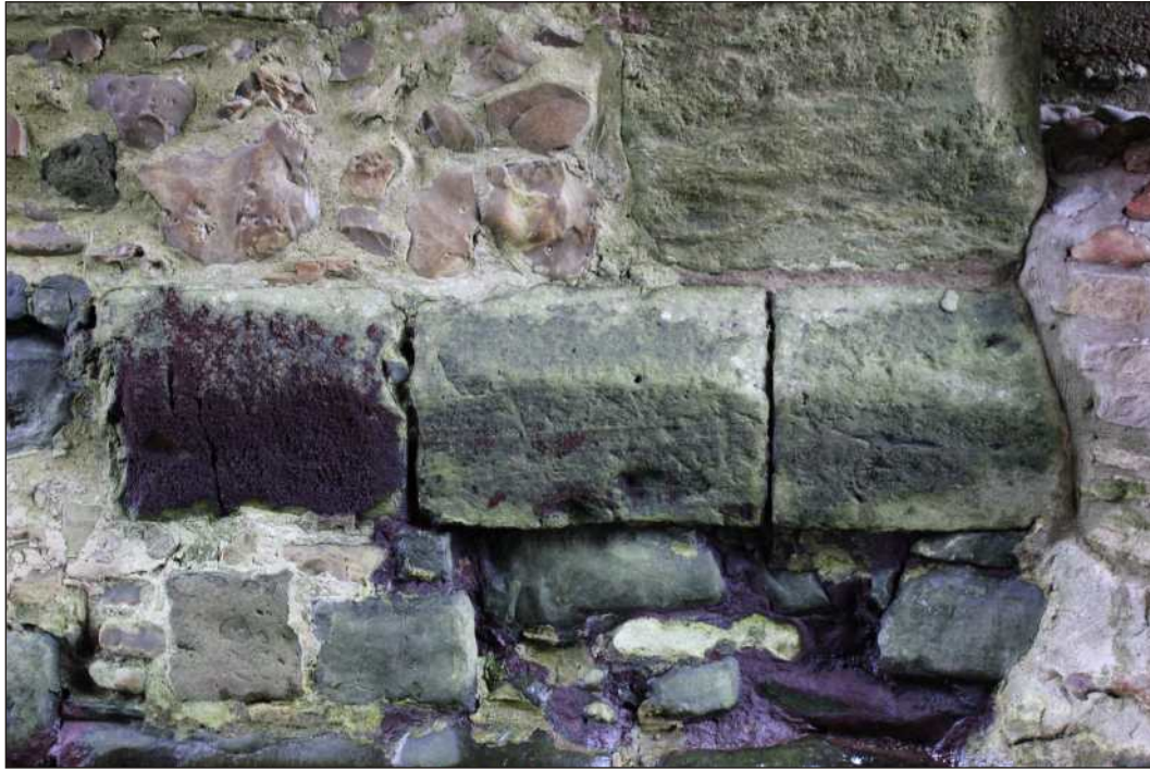
Plate 5: Three chamfered stones forming a projecting string course on the east side of the bridge
