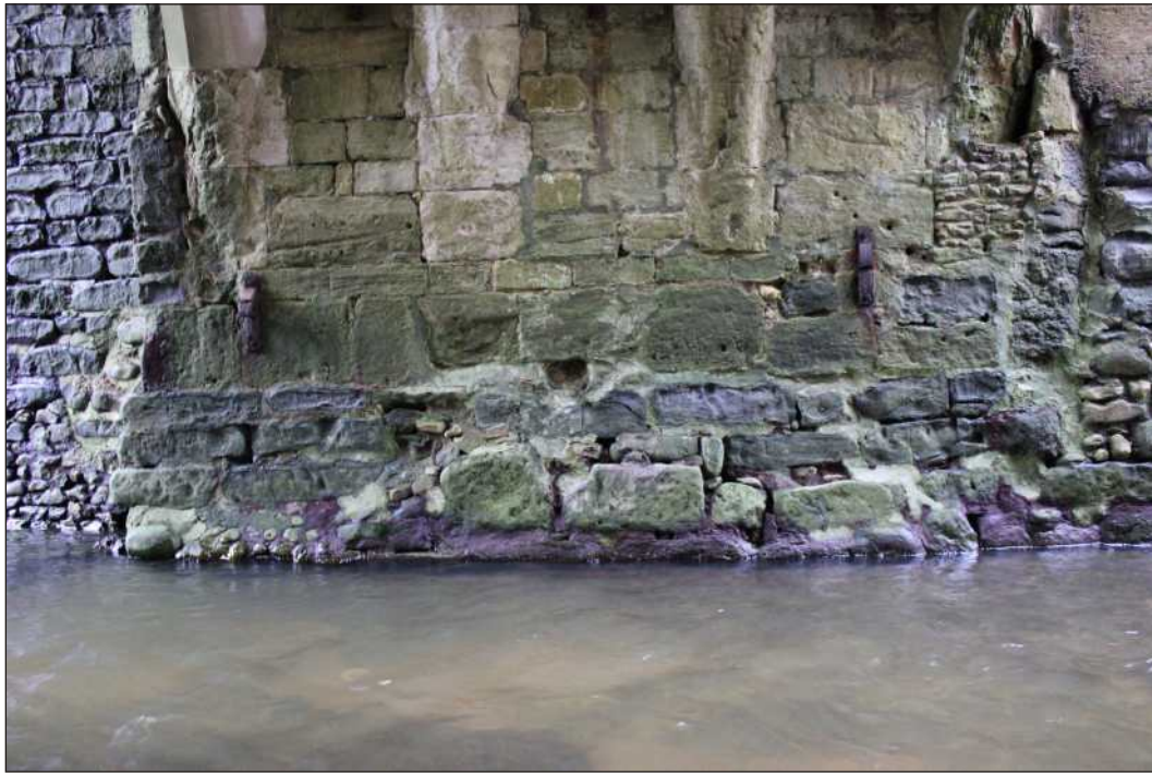
Plate 9: Lowest courses on the west side of the bridge
