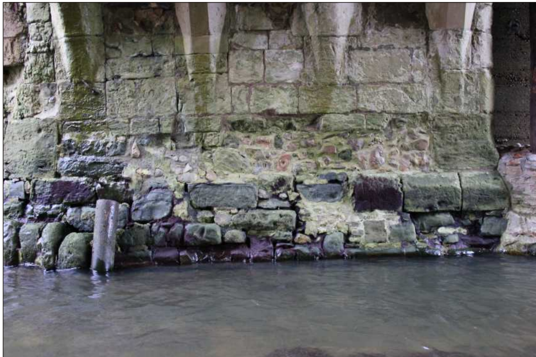
Plate 4: Lowest courses on the east side of the bridge
