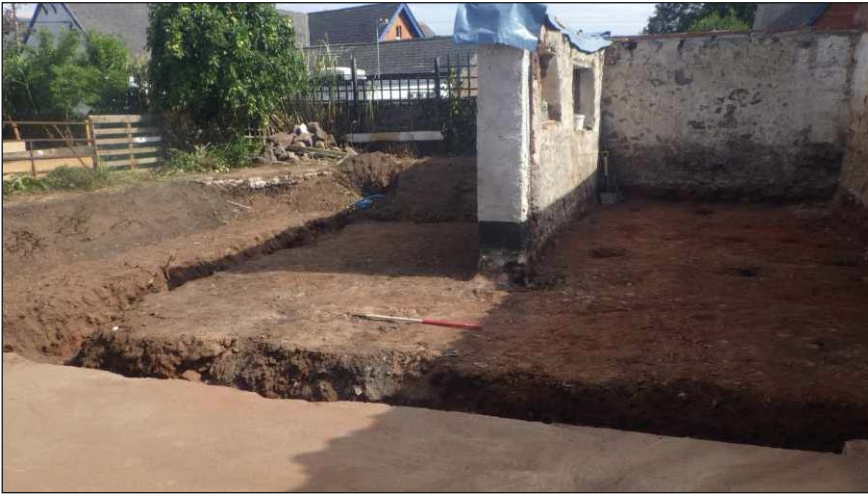
Plate 1: General view of site looking southeast (scale 1m)
