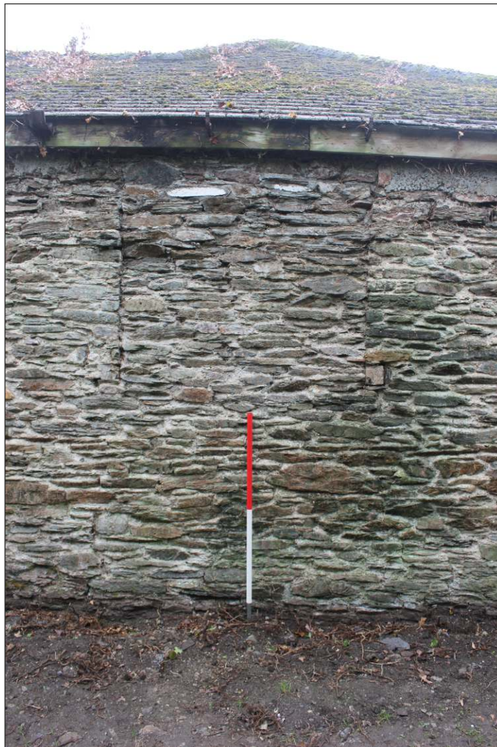
Plate 4: East external elevation showing blocked window, looking west. 1m scale
