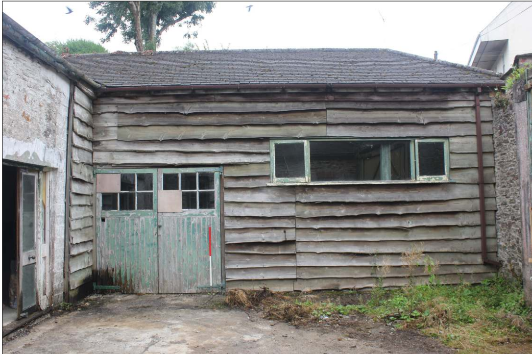
Plate 9: East range, west elevation, looking east. 1m scale
