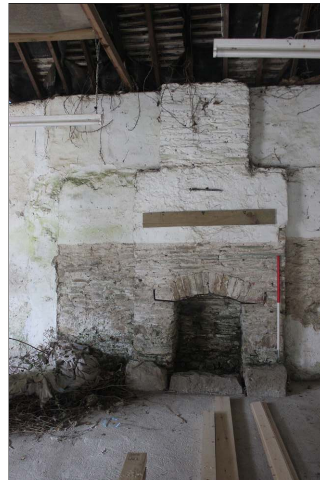
Plate 17: North range, fireplace in north elevation, looking north. 1m scale
