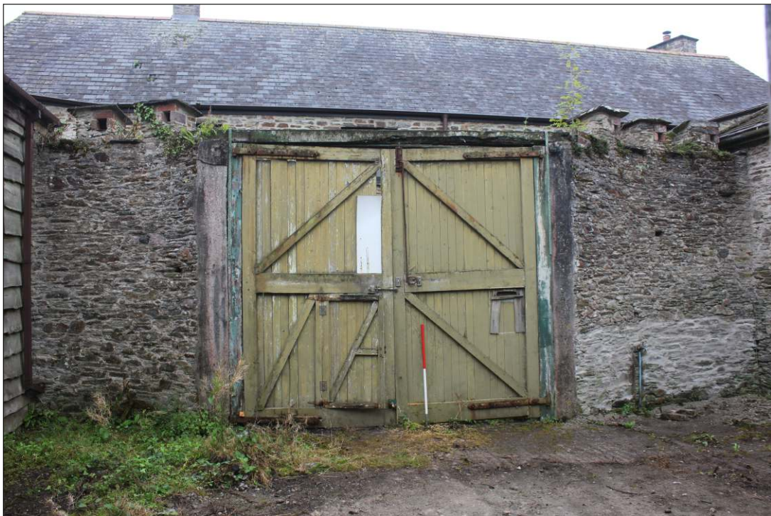
Plate 2: South wall of yard, looking south. 1m scale
