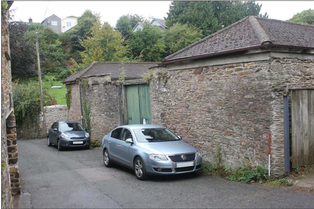
Plate 1: South external elevation, looking northwest. 1m scale
