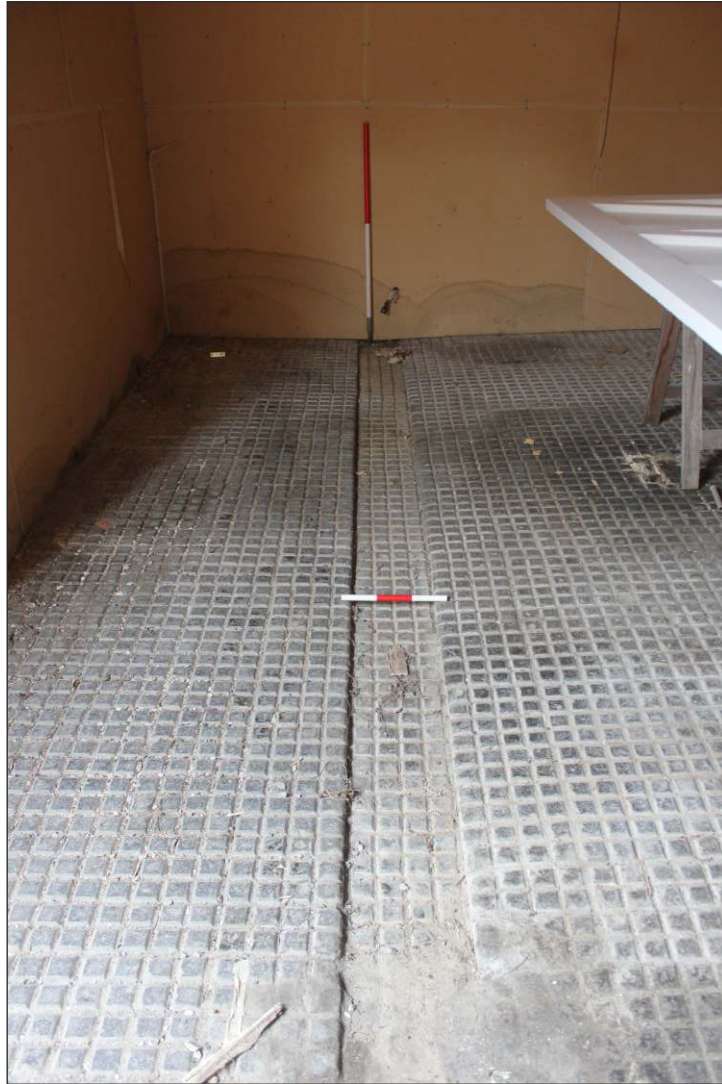
Plate 13: North range, west room drain, looking west. 1m and 0.30m scales
