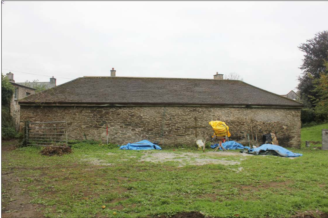
Plate 5: North external elevation, looking south. 1m scale
