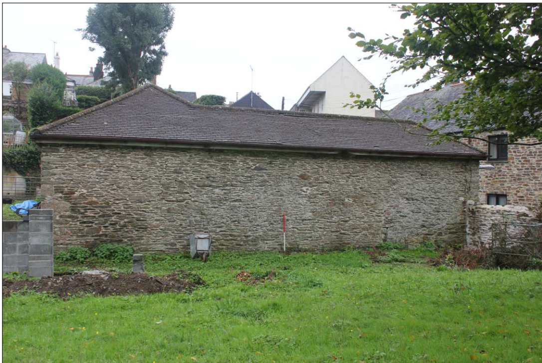
Plate 6: West external elevation, looking east. 1m scale
