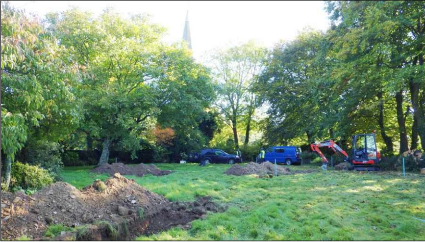
Plate 1: General working view of cable trench works looking west
