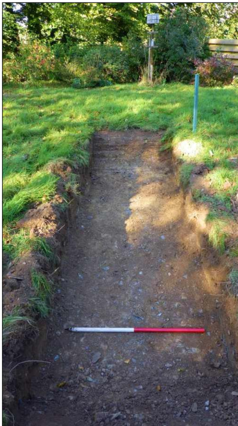
Plate 2: Excavated cable trench, view to northwest (scale 1m)
