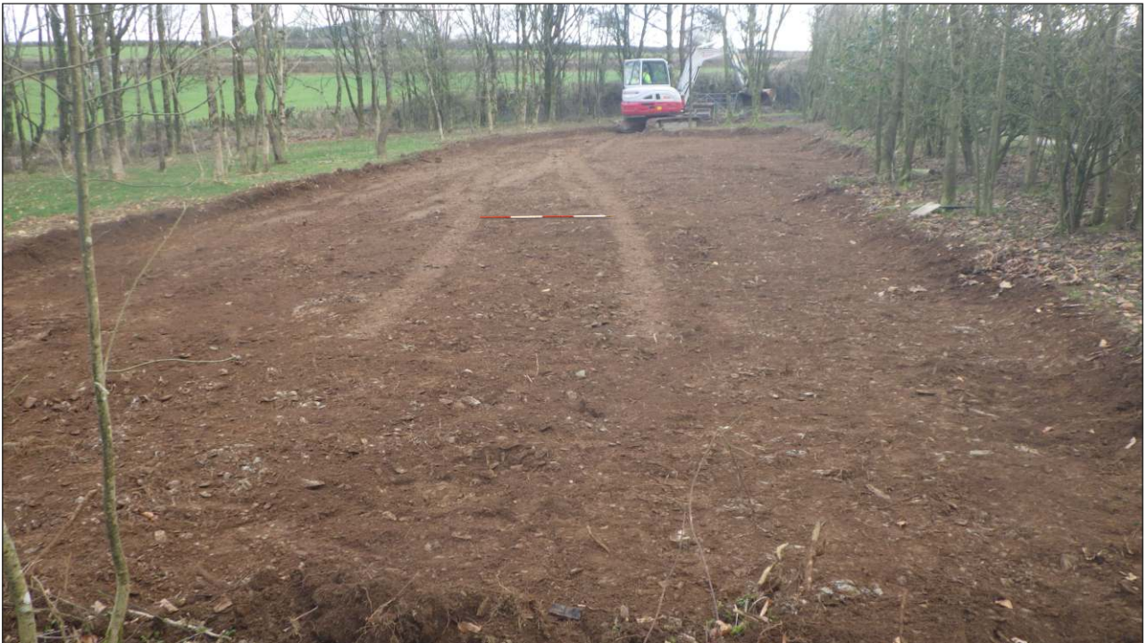
Plate 1: The footprint of the building looking east-northeast (2m scale)
