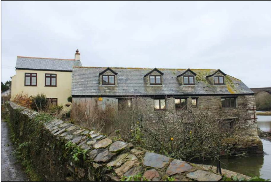
Plate 1: The tide mill, with mill house to the left, looking north
