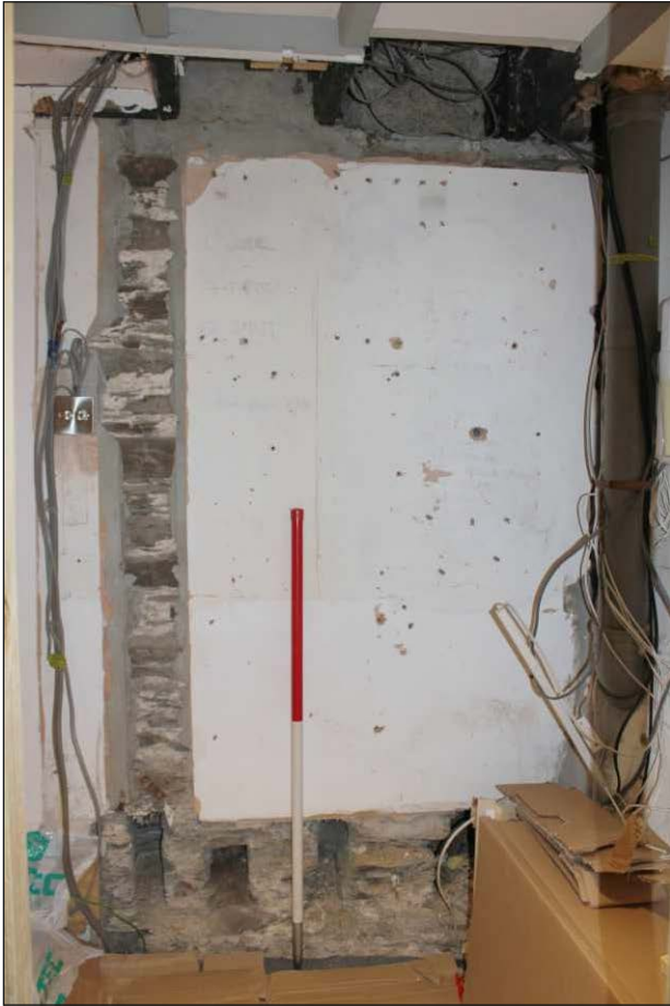
Plate 5: The interior wall of the tide mill prior to removal of finishes, looking southwest (1m scale). Joist sockets are visible at the base of the wall
