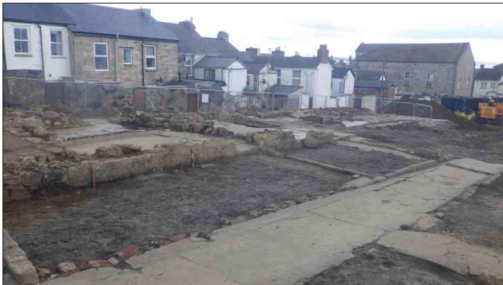
Plate 2: General view of the site showing Camberwell Street (foreground) with houses 8-11 to the rear as well as the front gardens of houses 10 and 11, looking east. 0.40m scale
