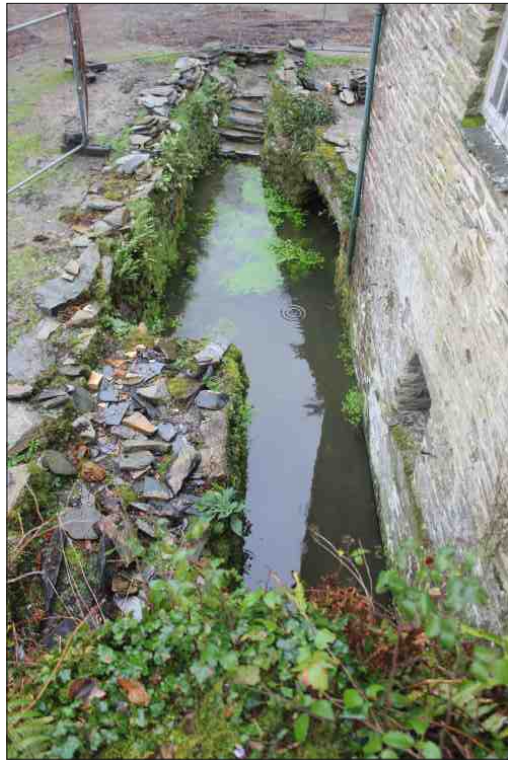
Plate 10: The north wheelpit, looking east
