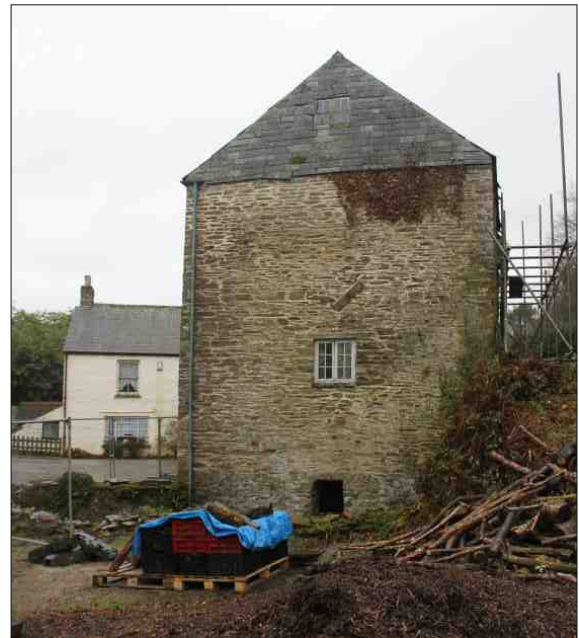
Plate 6: The north elevation, looking south
