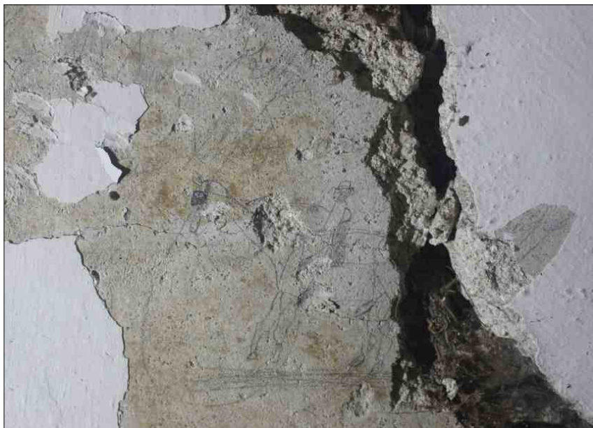
Plate 23: Horse and rider graffiti on south wall of the third floor, looking south
