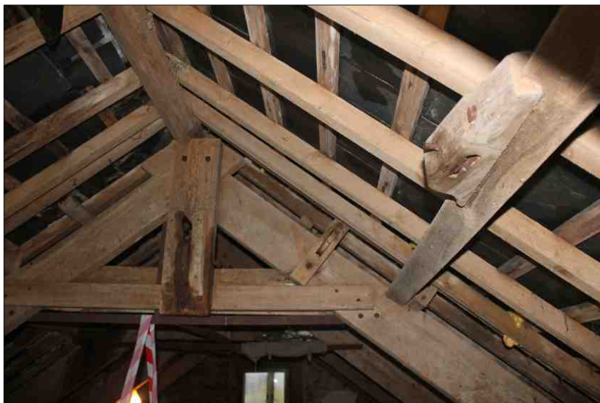
Plate 24: Pulleys for sack hoists on the third floor, looking south
