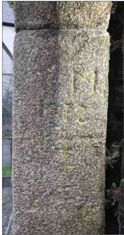
Plate 4: Graffiti on south jamb in east elevation doorway, looking south
