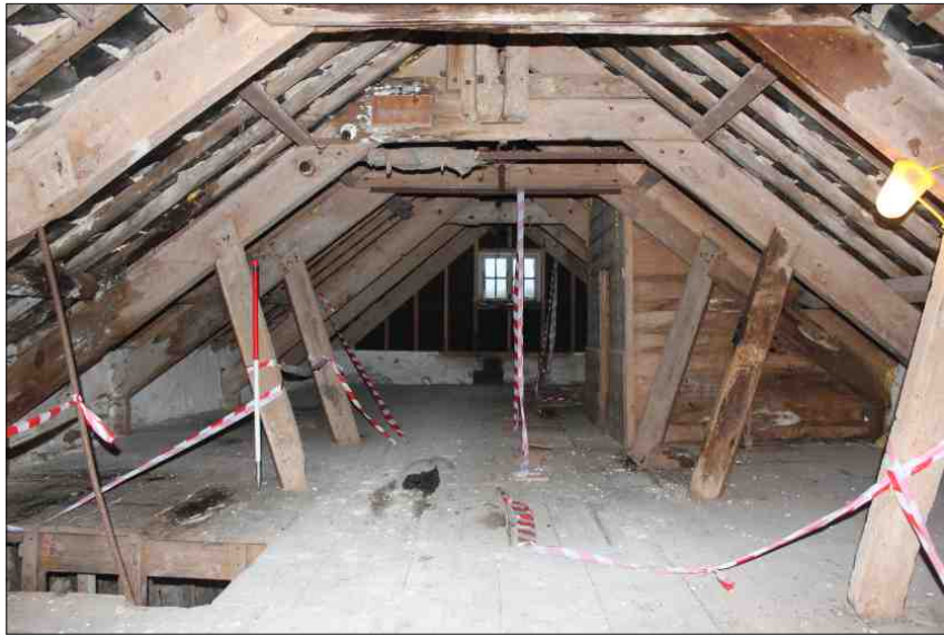
Plate 22: General view of the third floor, looking north (1m scale)
