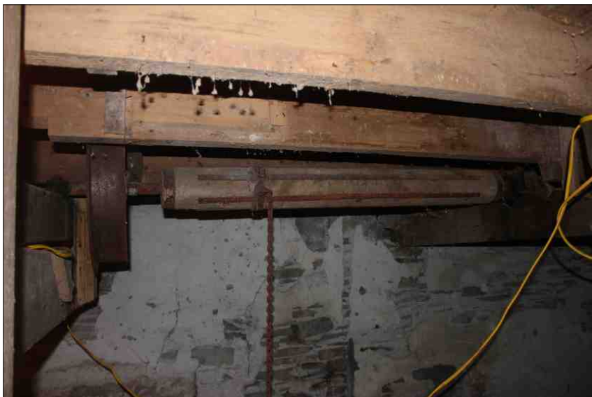
Plate 21: View of wooden roller and belt drive at northern end of second floor, looking north
