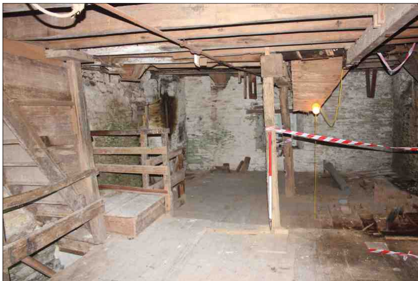
Plate 14: General view of the first floor, looking north (1m scale)
