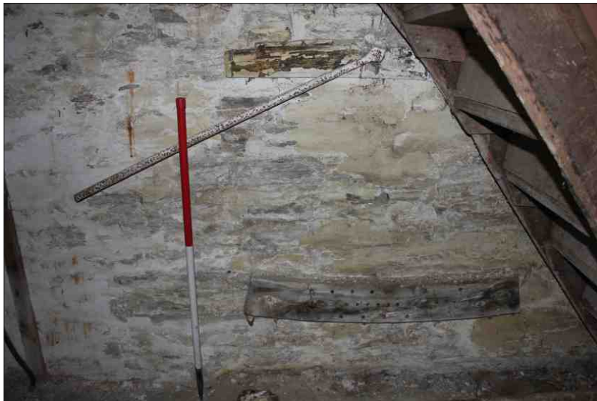
Plate 17: View of penstock control gear and peg board, looking west (1m scale)
