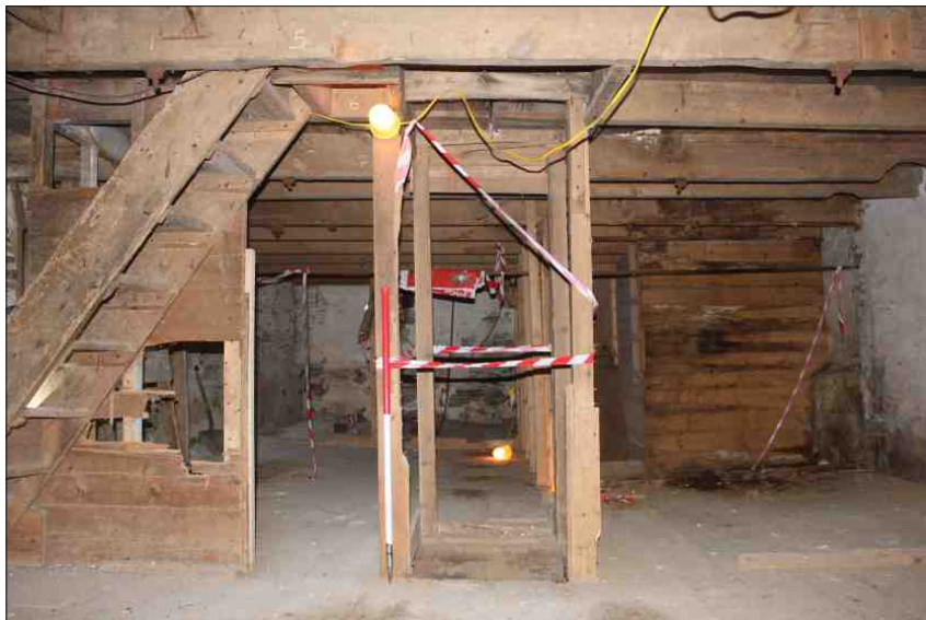
Plate 18: General view of the second floor, looking north (1m scale)
