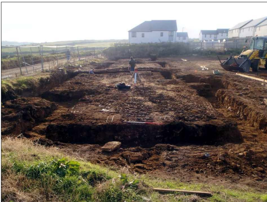
Plate 2: General view of foundation trenches, looking southeast (1m scale)
