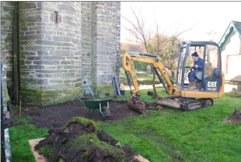
Plate 2: Showing groundworks in progress. View to southwest
