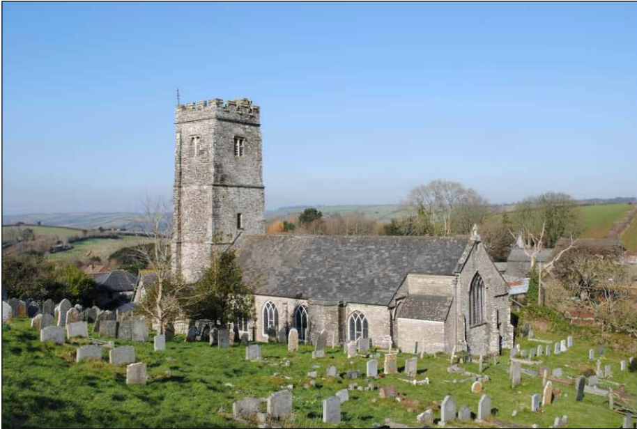
Plate 1: Church of St Peter, Cornworthy, looking northwest
