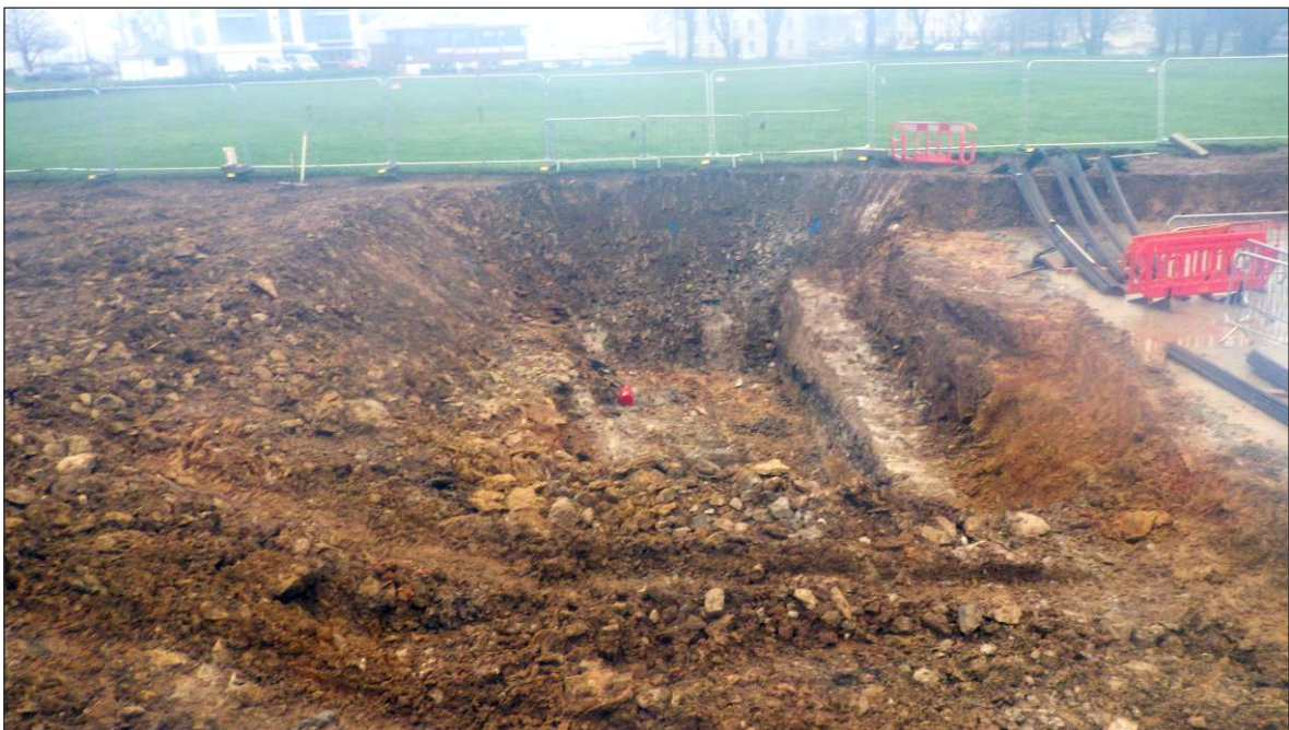
Plate 6: The Dock Lines ditch (part backfilled) during bulk reduction, looking southwest
