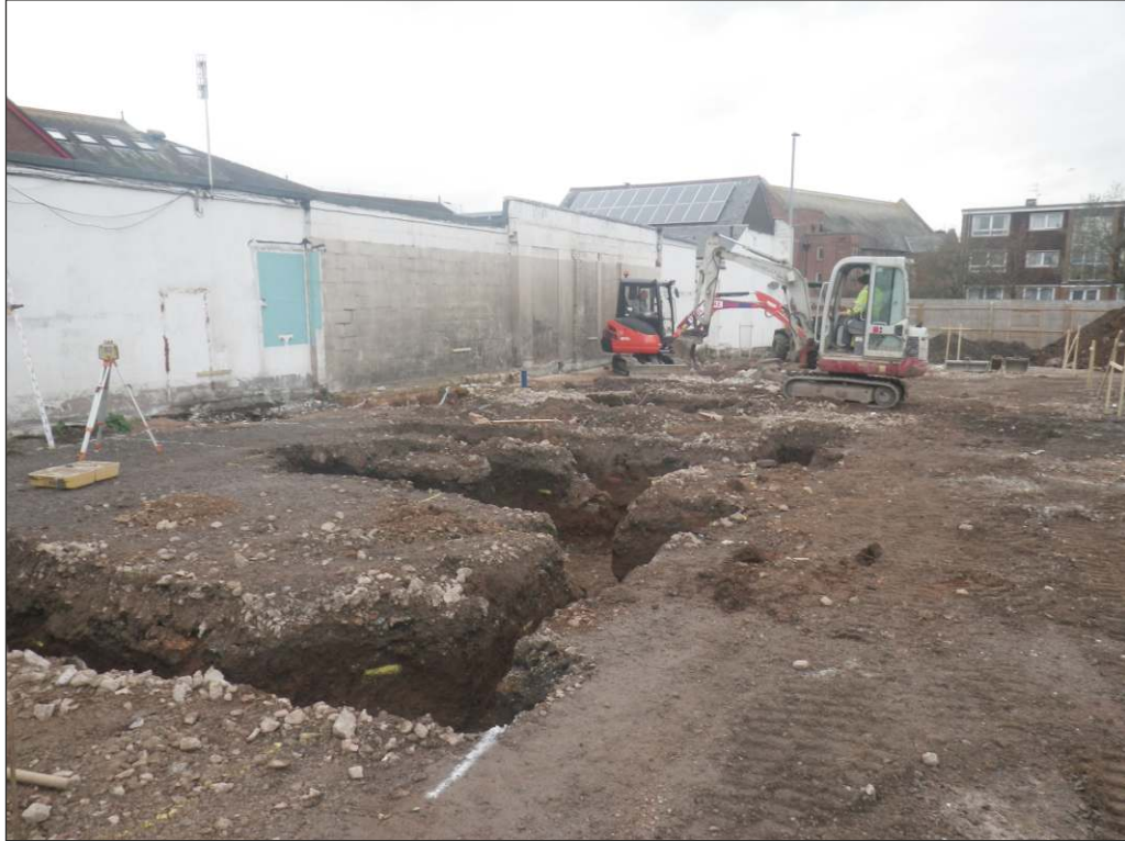
Plate 1: View of site during footings excavation. Looking northwest towards Cowick Street
