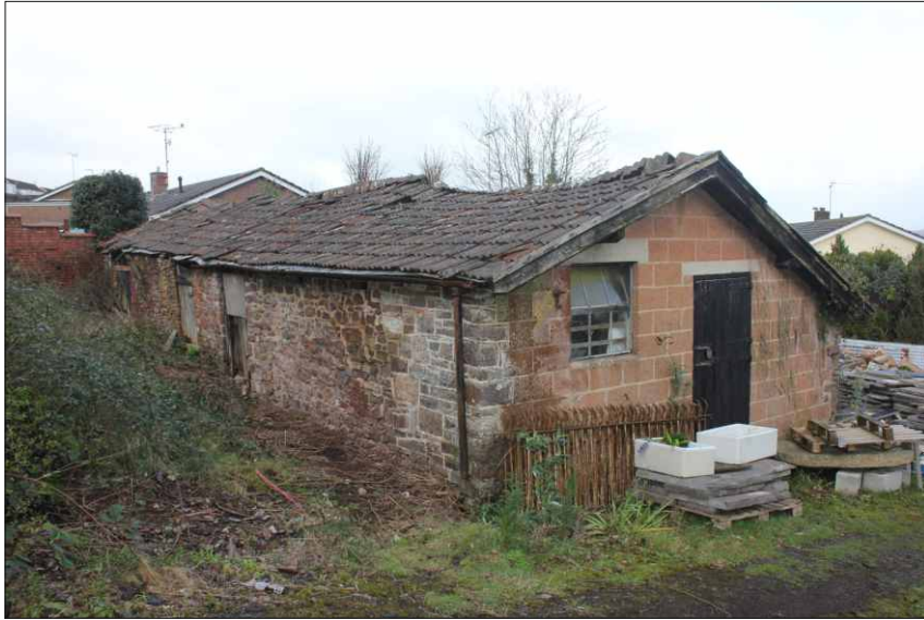
Plate 10: Unit 5, the south elevation and fully rebuilt east elevation, looking northwest
