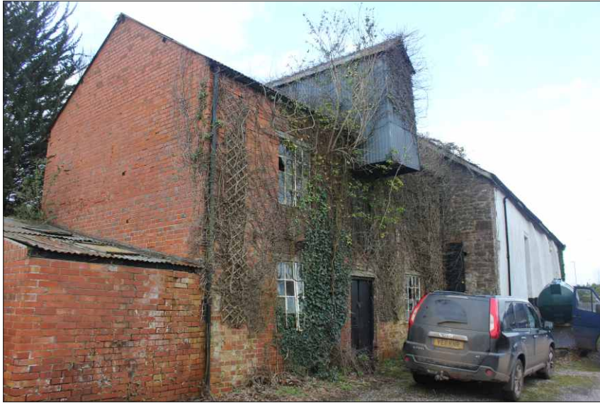
Plate 1: Unit 1, the north elevation, with Units 2-3 beyond, looking southwest
