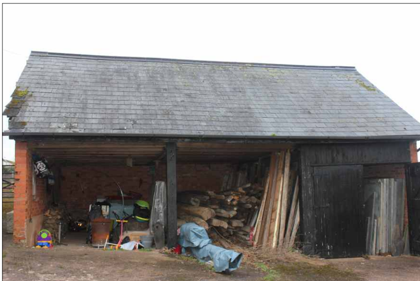
Plate 9: Unit 5, the east elevation, looking northwest
