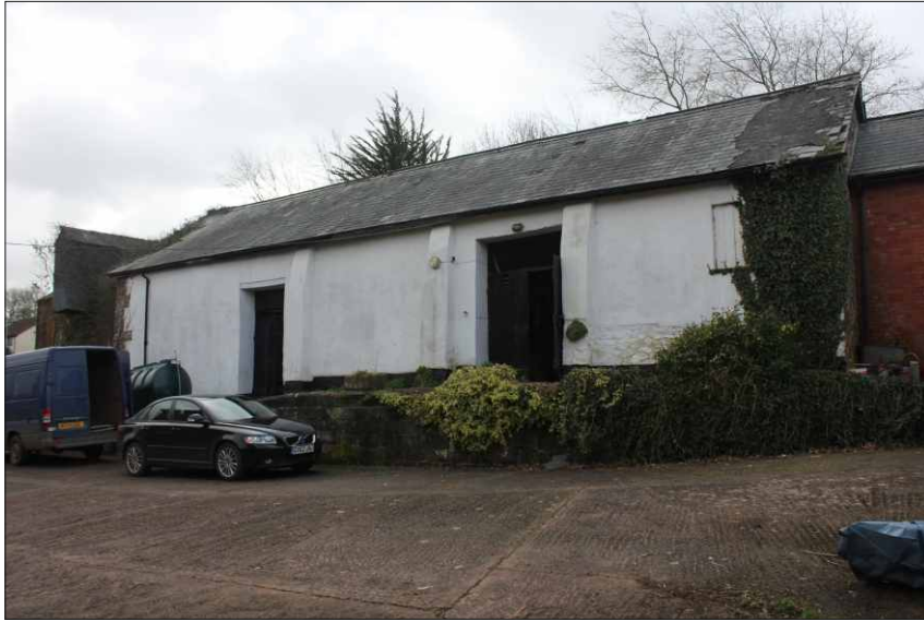
Plate 4: Units 2-3, the north elevation, looking southeast
