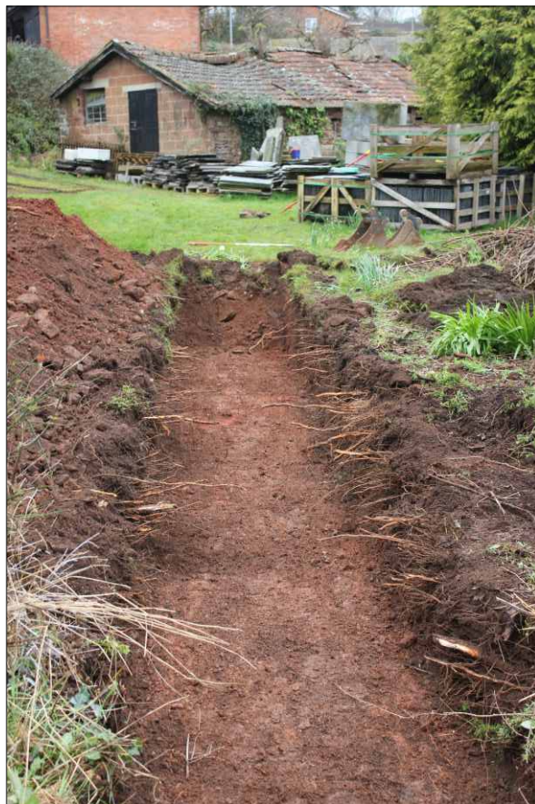
Plate 15: Trench 1, looking southwest. 1m scale
