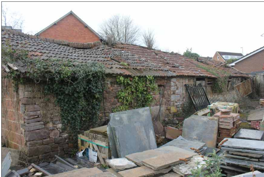
Plate 11: Unit 5, the north elevation, looking southwest
