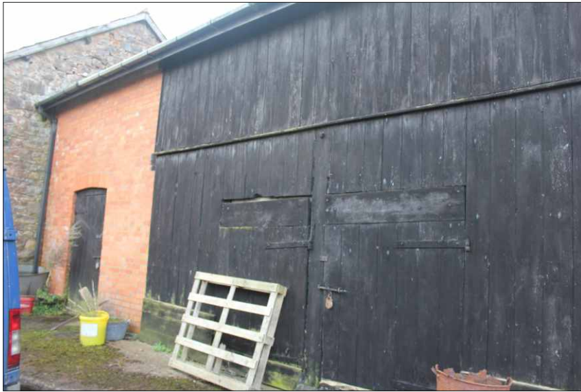
Plate 7: Unit 4, the north elevation, looking south
