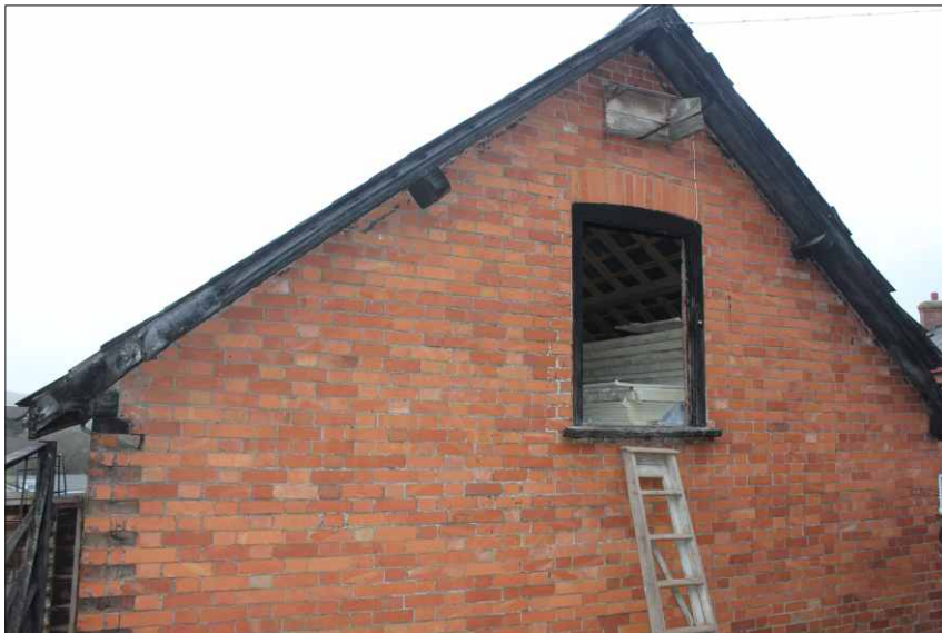
Plate 8: Unit 5, the south elevation showing the first-floor access and scar of former boundary wall, looking north
