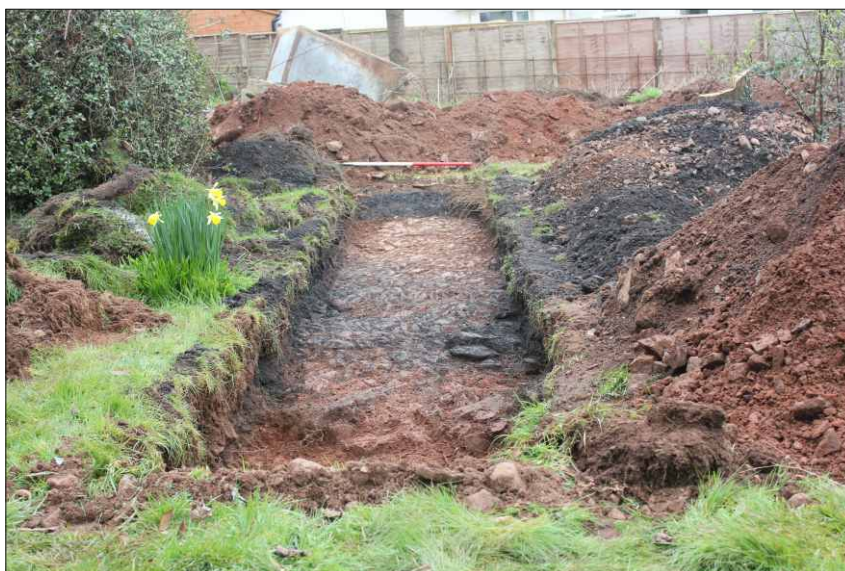
Plate 16: Trench 2, looking northwest towards trench 1. 1m scale
