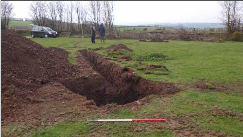
Plate 1: View of monitored excavations, looking southwest (1m scale)
