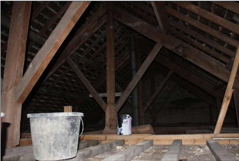
Plate 11: The roof structure, looking east
