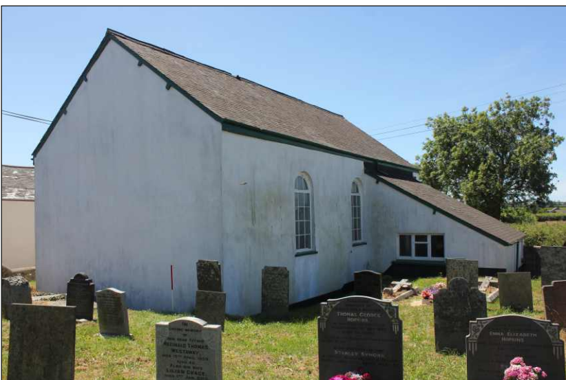
Plate 3: The east and north elevations, looking southwest (1m scale)
