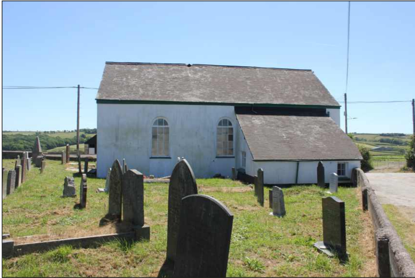
Plate 4: The north elevation and north extension
