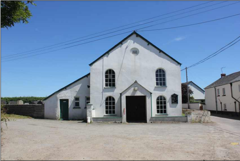
Plate 1: The west elevation, looking east (1m scale)
