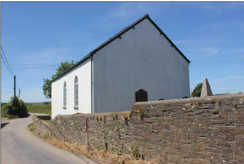
Plate 2: The south and east elevations, and south boundary wall, looking northwest (1m scale)
