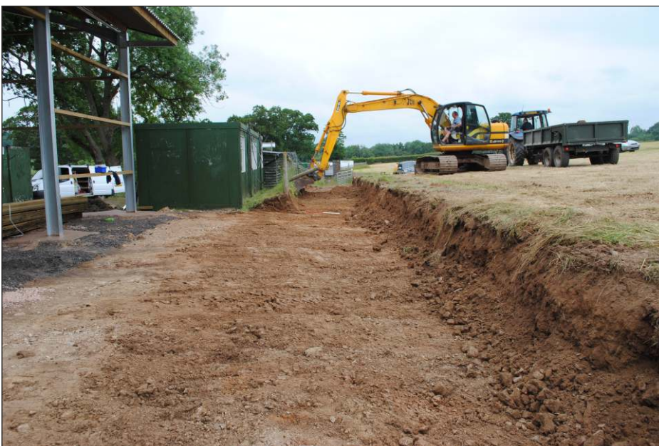
Plate 3: View of groundworks extension, work in progress, looking northeast
