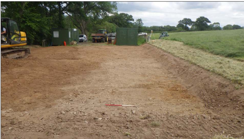
Plate 2: View of the groundworks, looking northeast 1m scale
