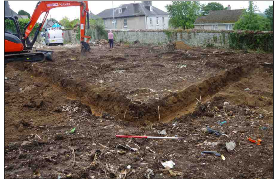
Plate 2: View of trench, looking southeast (1m scale)
