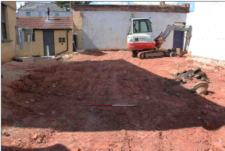
Plate 2: General view of the stripped area, looking southwest (1m scale)
