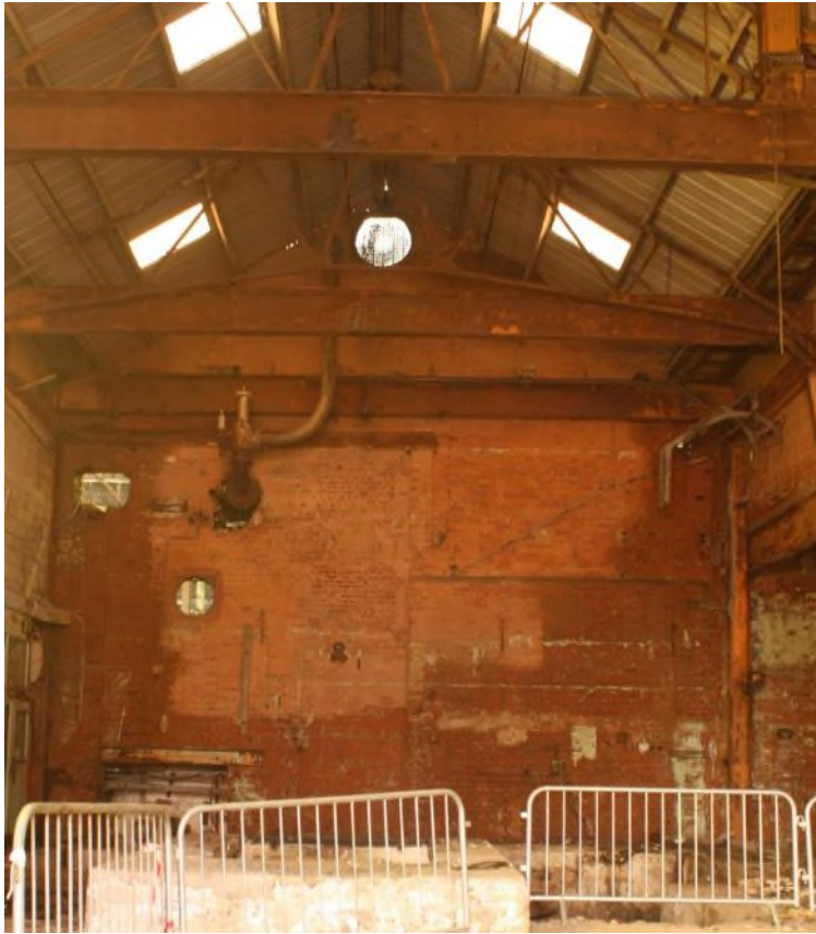
Building 20, Power house, interior, west part facing north (9542)
