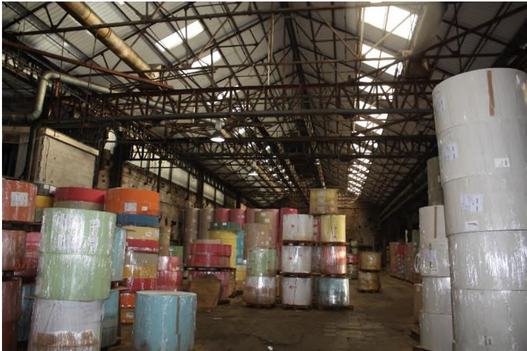
Building 23 Interior. General view looking south-east. (8303)
