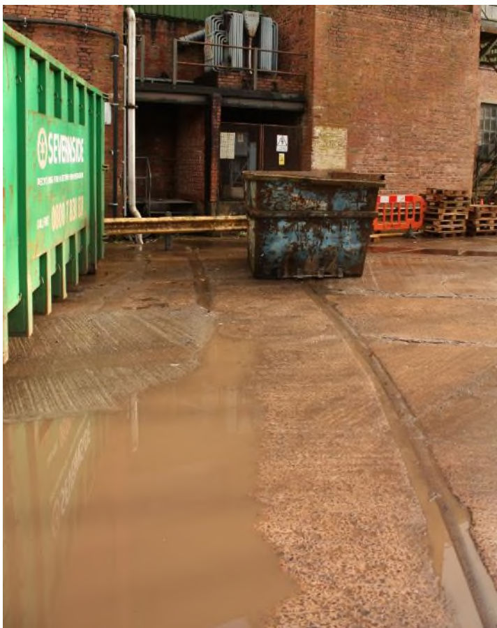
Rail tracks to the west of Buildings 3 and 4 leading towards the Tunnel Passage between Bdg.3 and Bdg.6. (8290)
