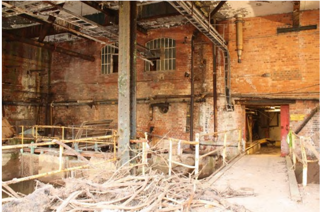
Building 15 East elevation between the Power House (Bdg.20) to the south and the Pump House (Bdg. 17) to the north (out of shot). The Leat/Headrace (18) is the covered area to the left of the picture.
