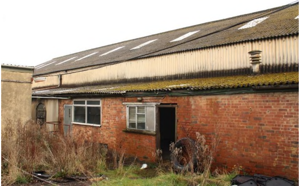
Building 30 West elevation facing north-east. (8375)
