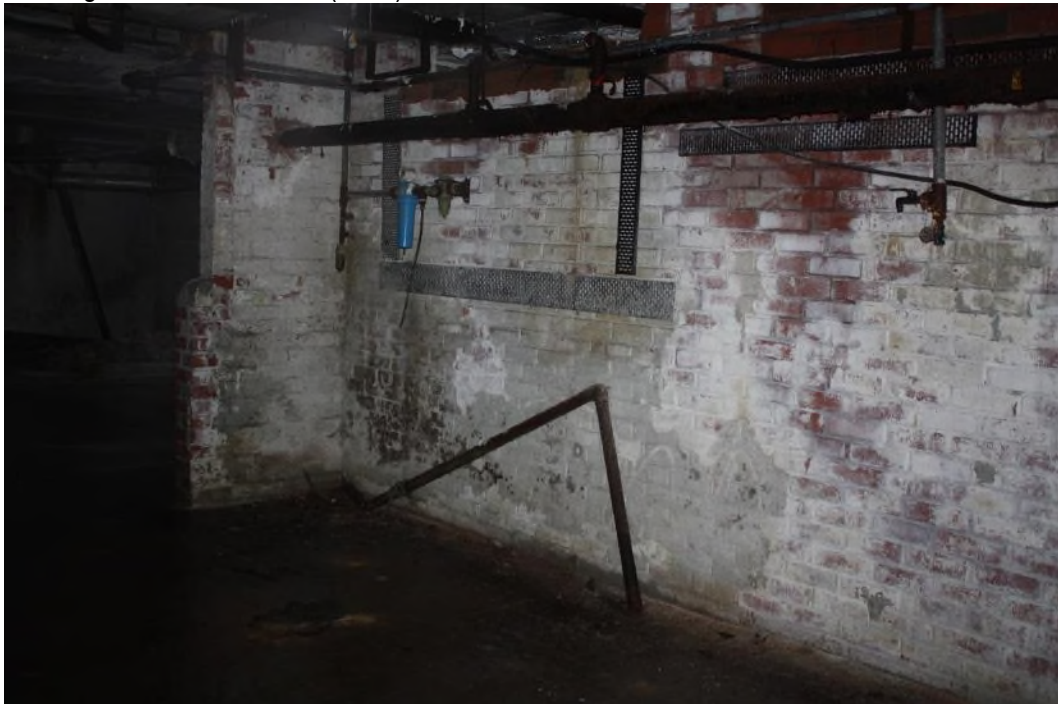
Building 12 Interior looking south-west. (8122)
