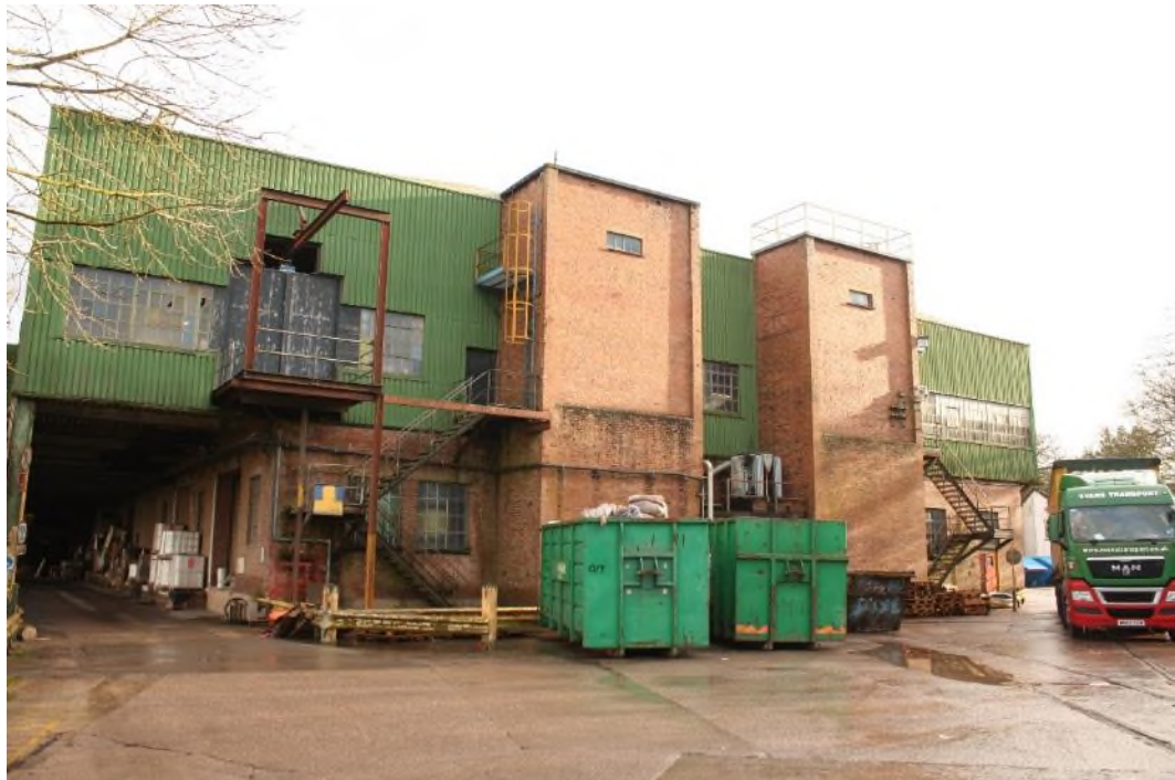
Buildings 3 (left) and 4 (right), west elevation with the covered way along the north side of Building 3. (8288)
