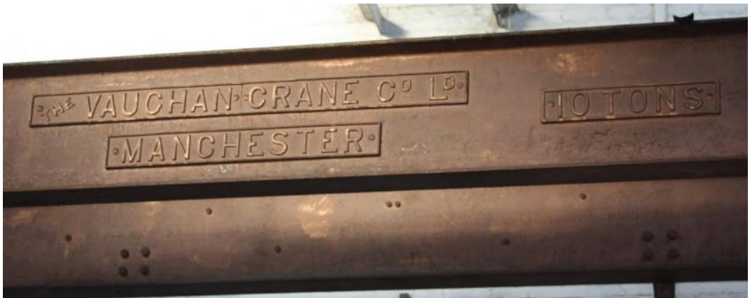
Building 28 Travelling hoist manufacturer's name in iron beam.
