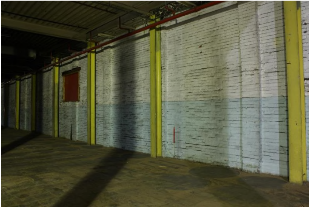
Building 3 Ground floor, south wall facing south-east. (9575)
