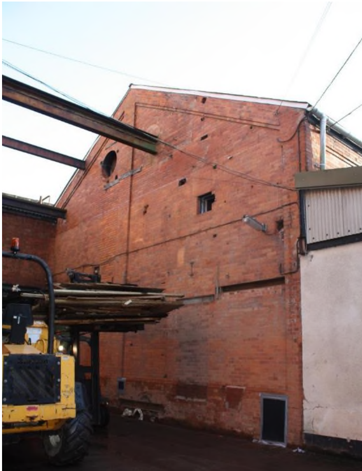
Building 28, north elevation facing south-east. (8360)
