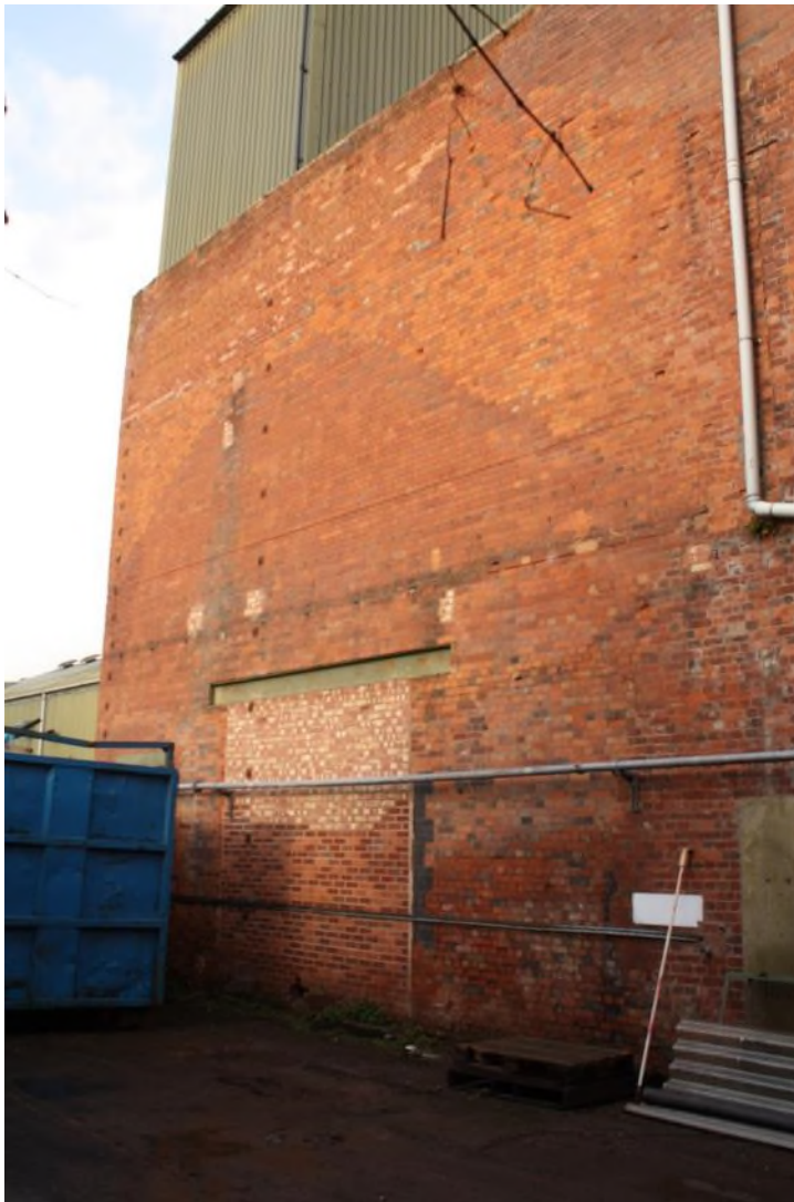
Building 22 Reactor House, south elevation, west part, facing north-west. (8337)
