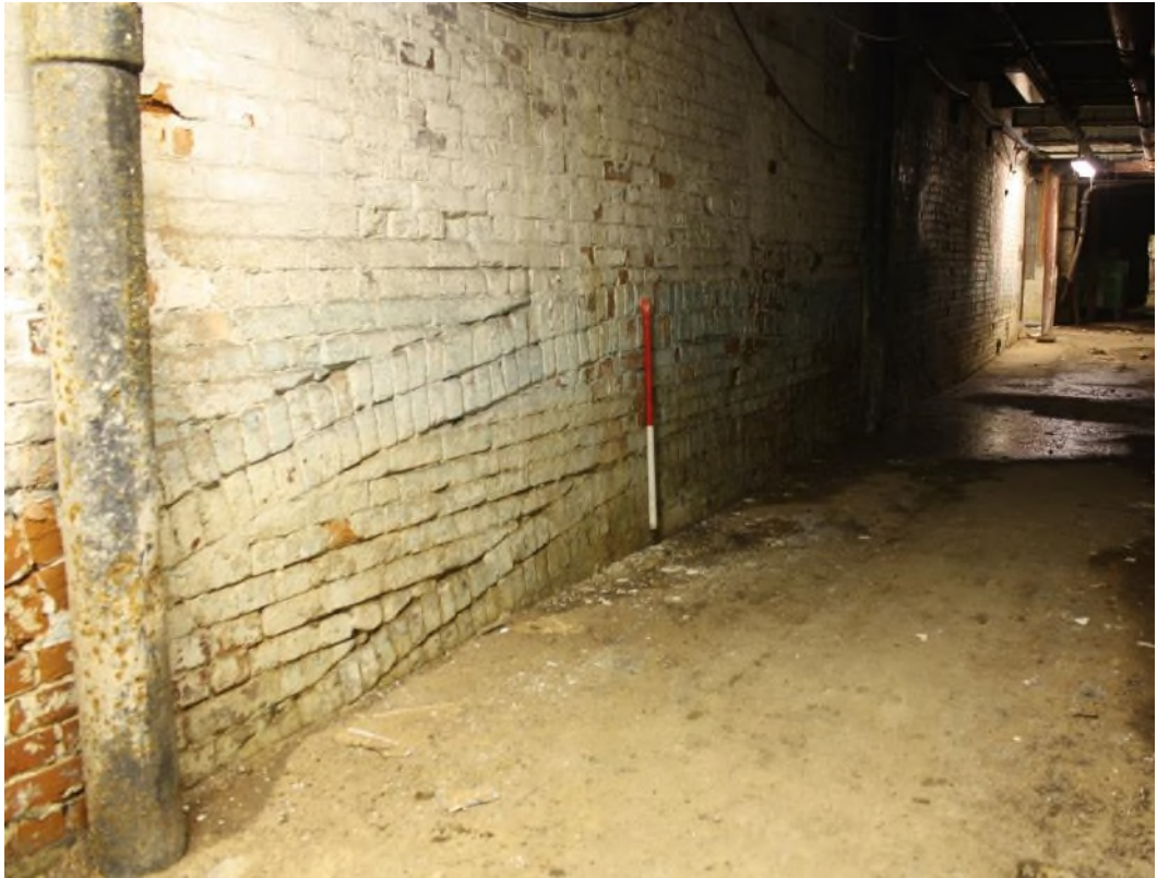
Building 16 South-east elevation, facing north showing the wide, low arch spanning the river. (9565)
