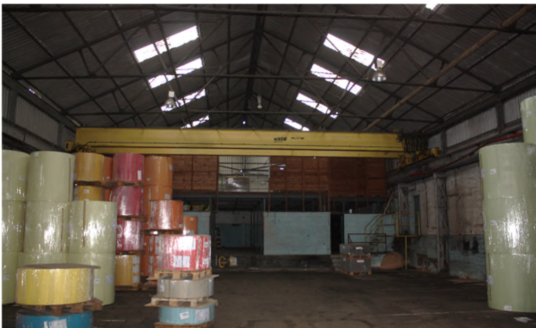
Building 30 Interior facing south. (8376)
