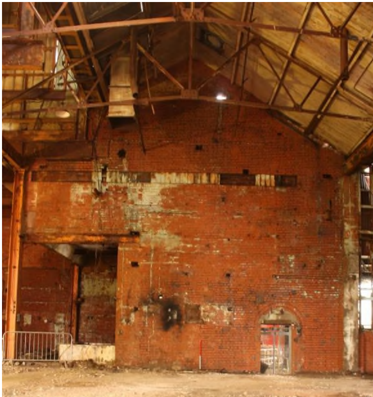
Building 20 Power House, interior east part facing north (9540)
