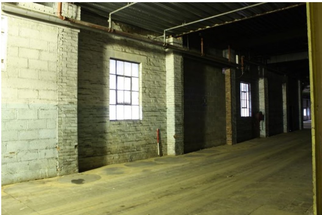
Building 3 Ground floor, north wall facing north-east. (9577)
