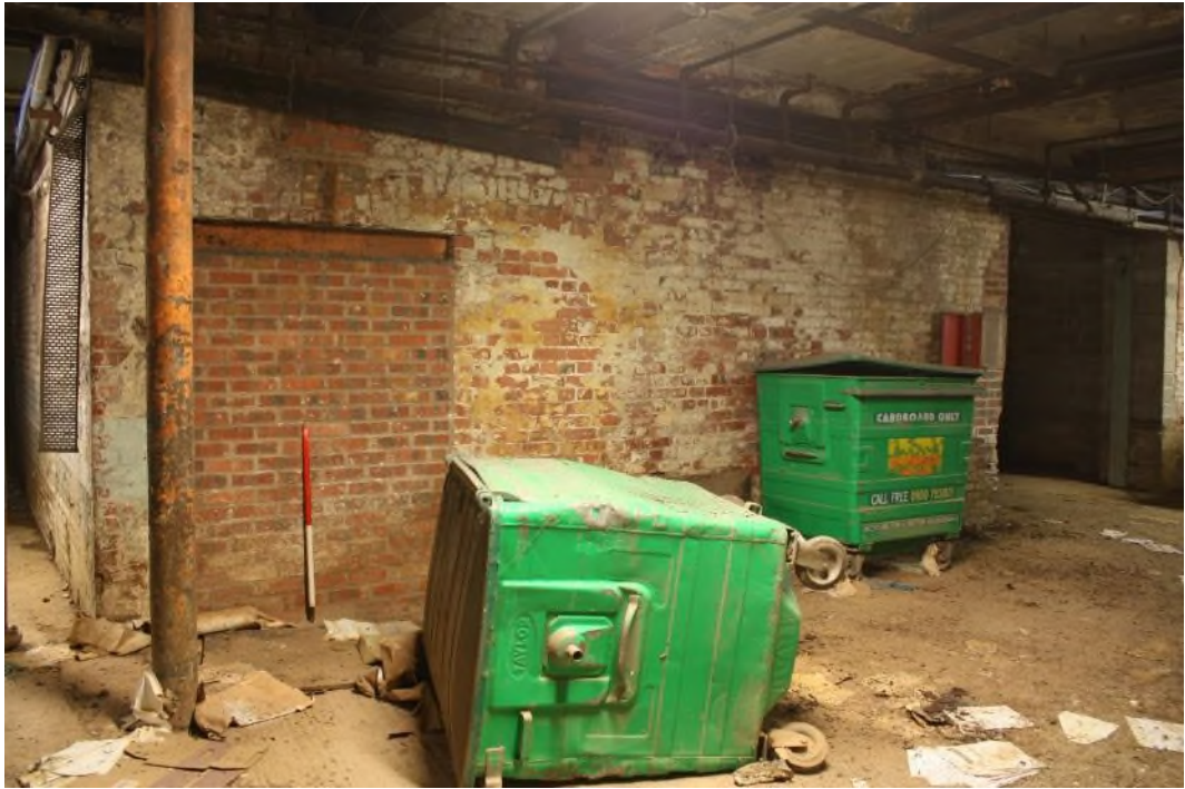
Building 16 North-east gable end, facing south-west. (9467)
