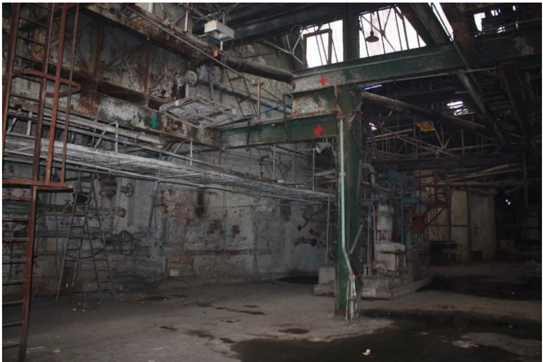
Building 15 General view at upper floor level facing north-west. (8234)
