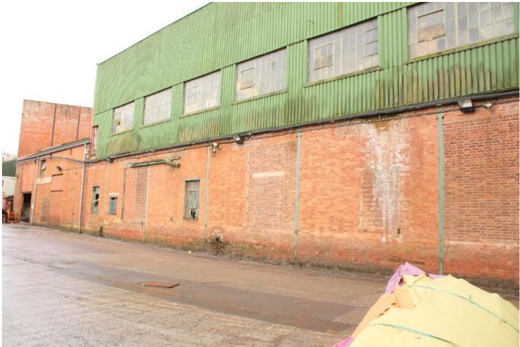
Building 3 North elevation, east part looking south-east. (8215)
