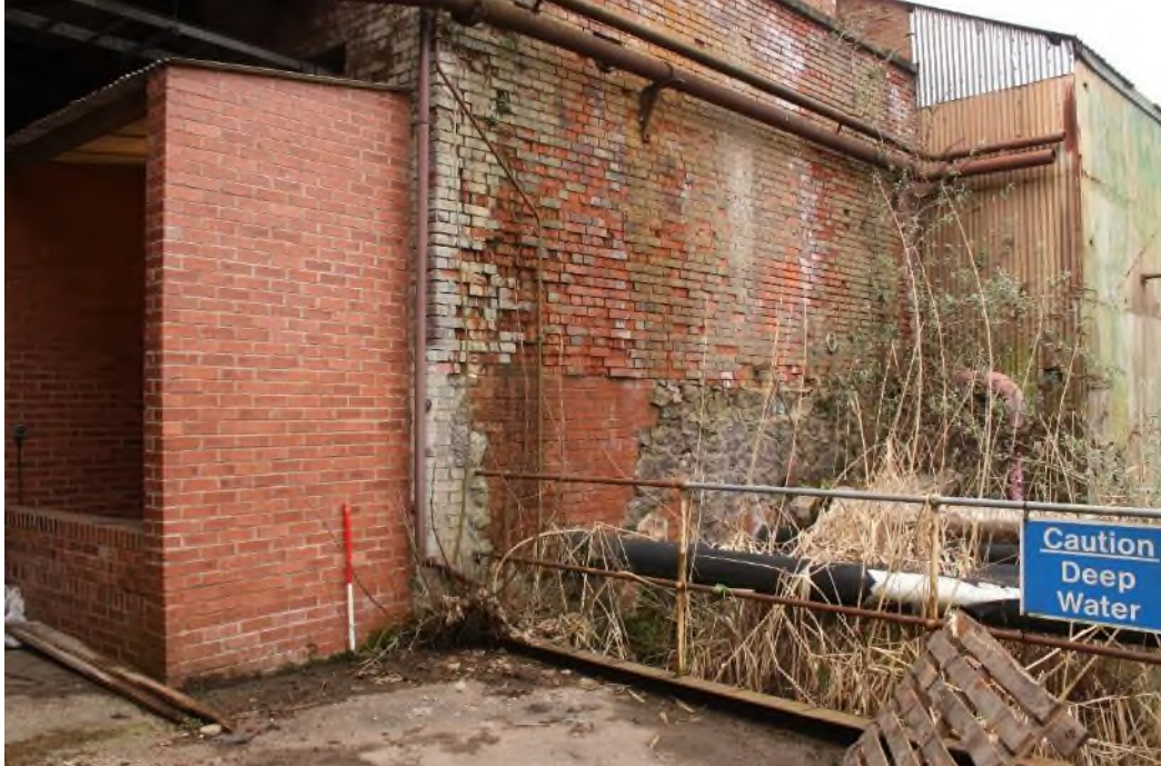
East elevation of the Pump House (Bdg.17) showing the lower section of stone rubble walling with brickwork to the south and above. (9532)
