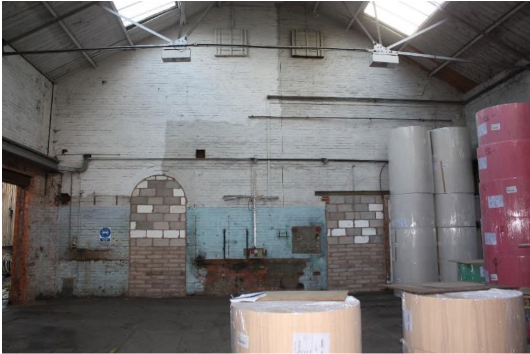
Building 28 Interior facing south. (8371)
