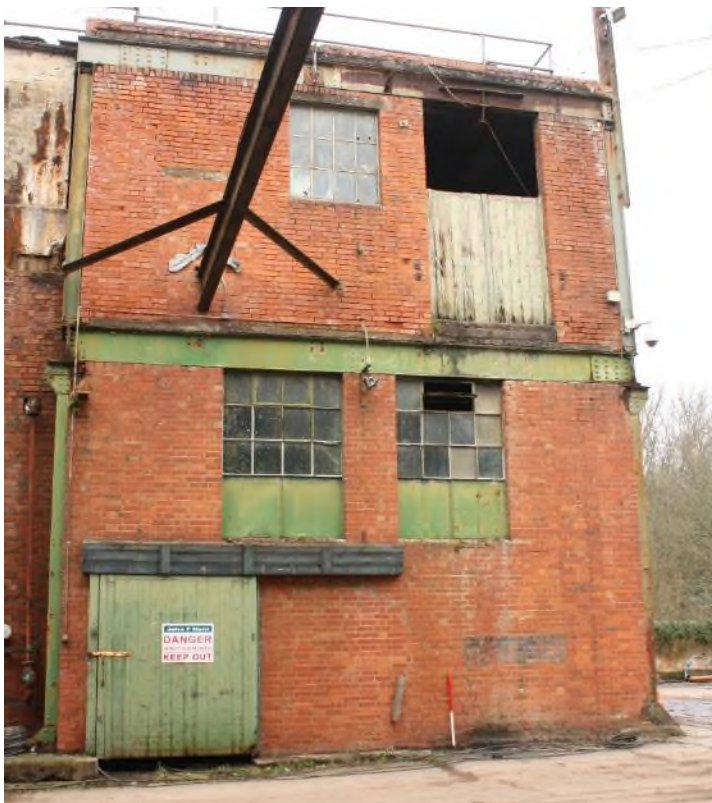
Building 19 Compressor Room, south elevation. (9535)
