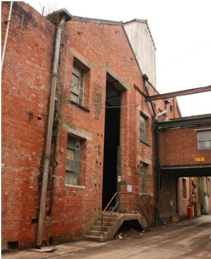
Building 20 Power House, south elevation, west part, facing north-east. (9543)
