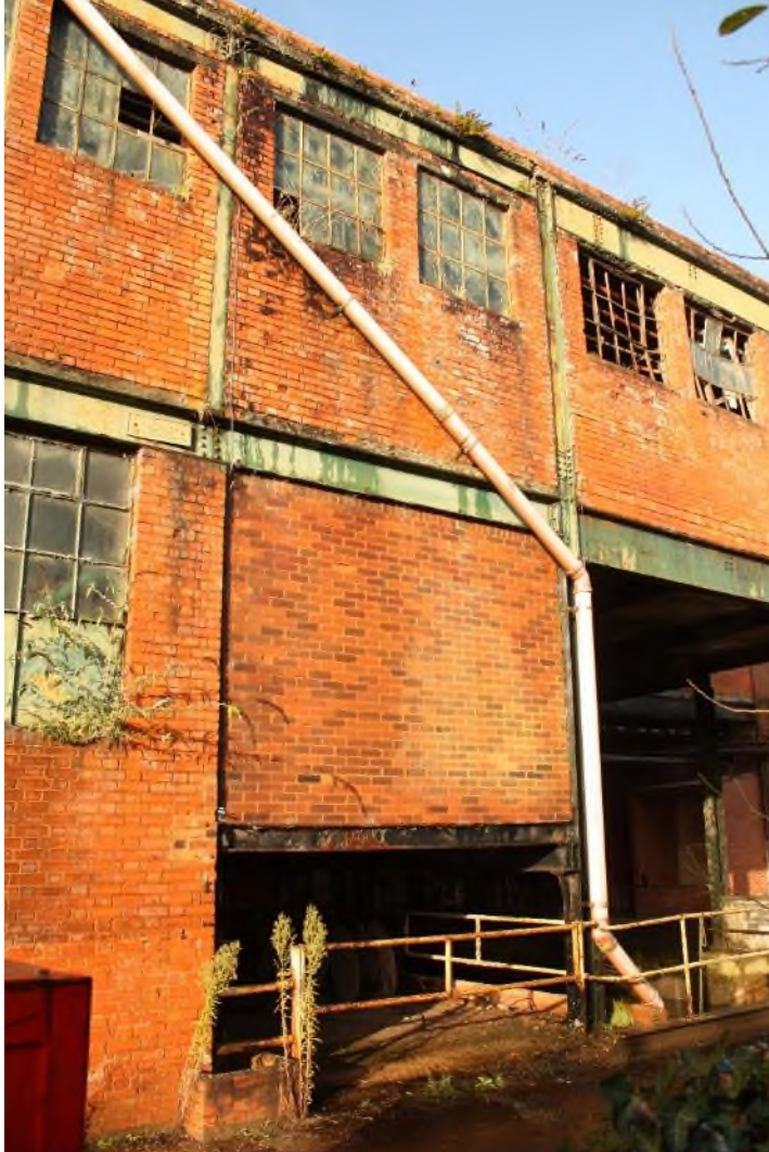
The east elevation of the building over the Leat/Headrace. (8084)
