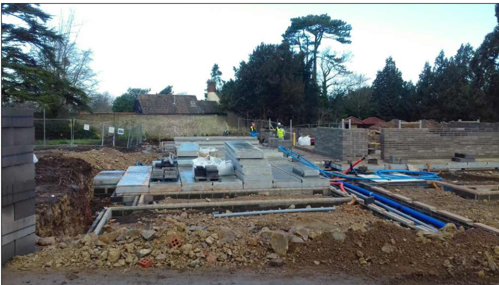
Plate 4: General view of construction in progress, looking northwest
