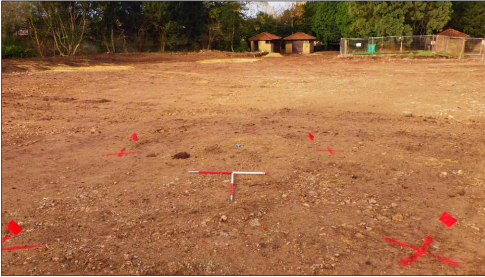
Plate 3: The levelled site, looking northeast (1m and 1m scales)
