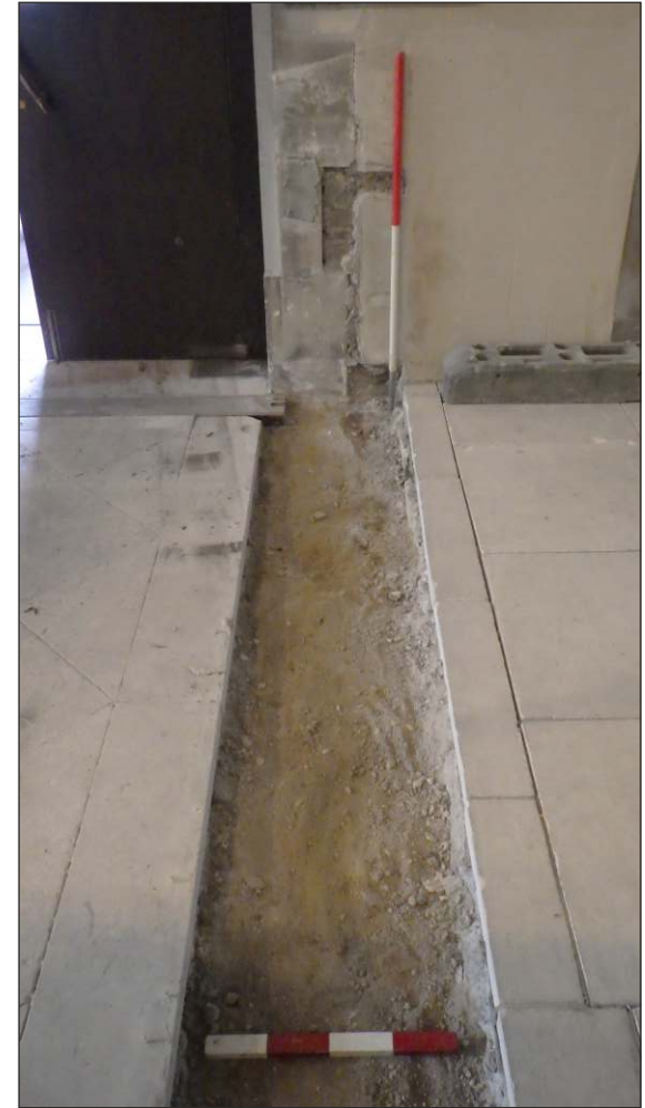
Plate 3: Showing removed wall scar. View to south (scales 1m and 0.4m)
