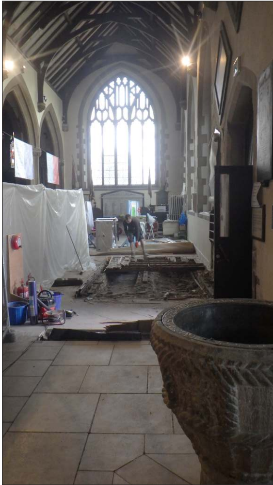
Plate 1: General working view looking east with Norman Font in foreground
