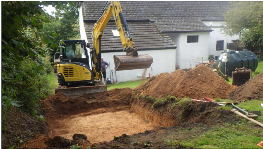
Plate 1: General working view of groundworks. Looking southeast towards 6 Newcourt Cottages.
