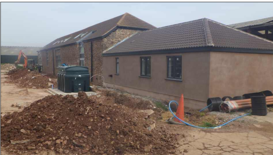
Plate 2: Working view of groundworks, looking north
