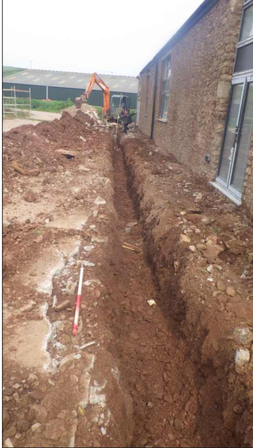
Plate 3: View of excavated trench, looking northwest (scale 1m)
