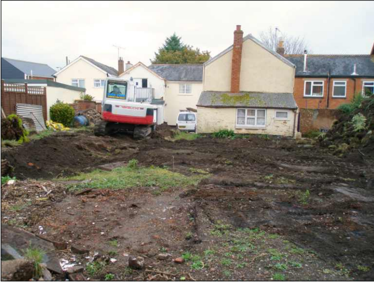
Plate 1: General view of site during topsoil stripping. Looking east
