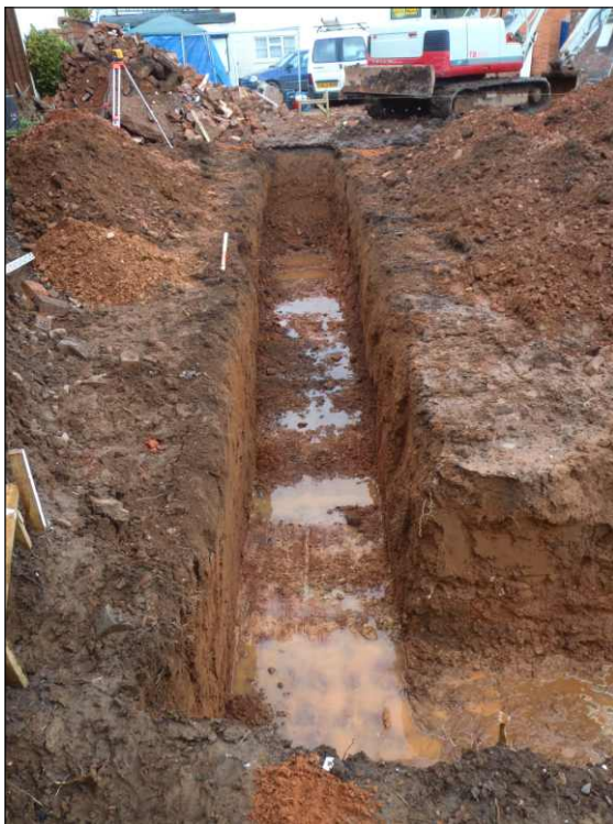
Plate 2: Working view of footings trench, looking east
