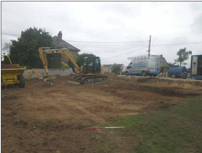
Plate 2: View of monitored groundworks, looking northwest (1m scale)
