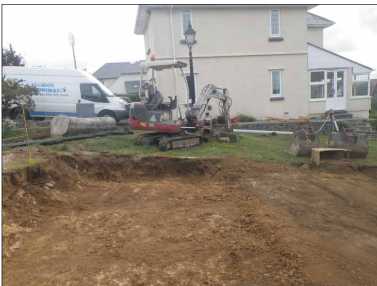
Plate 3: View of monitored groundworks, looking east (1m scale)
