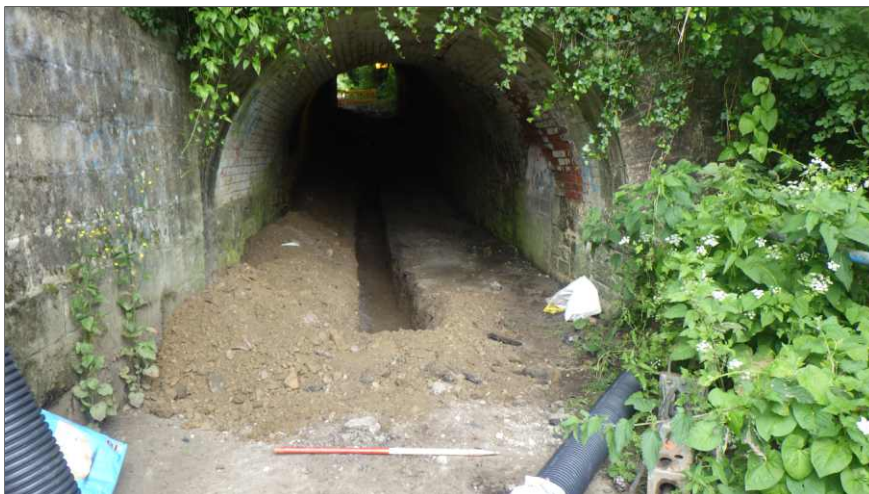
Plate 6: View of the trench within the tunnel, looking east (1m scale)
