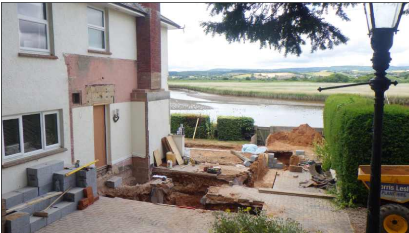
Plate 2: Showing excavated footings trenches. View to southwest (scale 1m)
