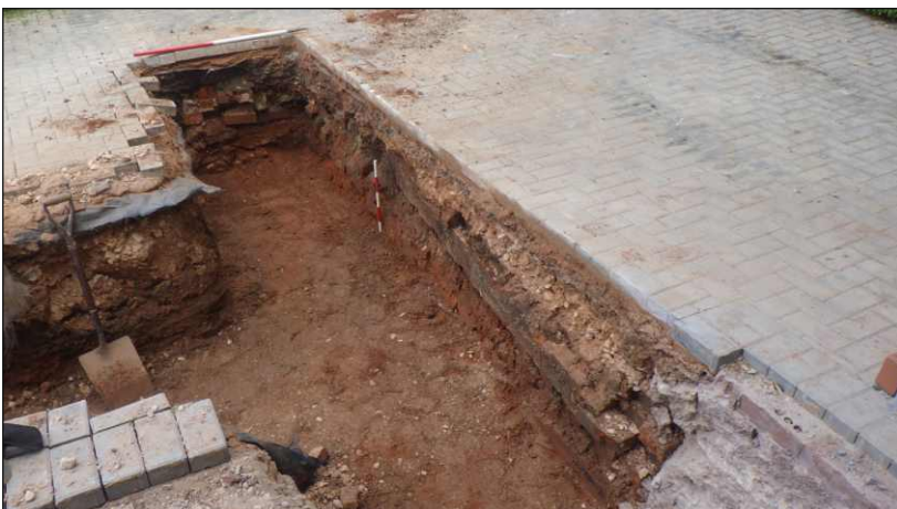
Plate 4: Showing excavated footing with brick footing S107. View to north (scale 0.5m)
