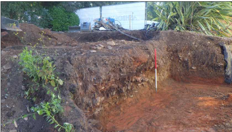
Plate 2: Showing terrace excavation. View to west (scale 1m)
