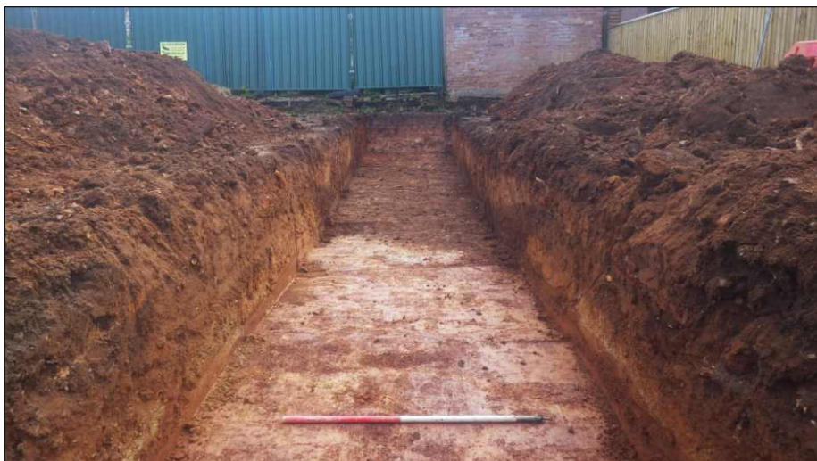
Plate 3: Trench 2, view to southeast with tree throw pit 104 in background (scale 1m)
