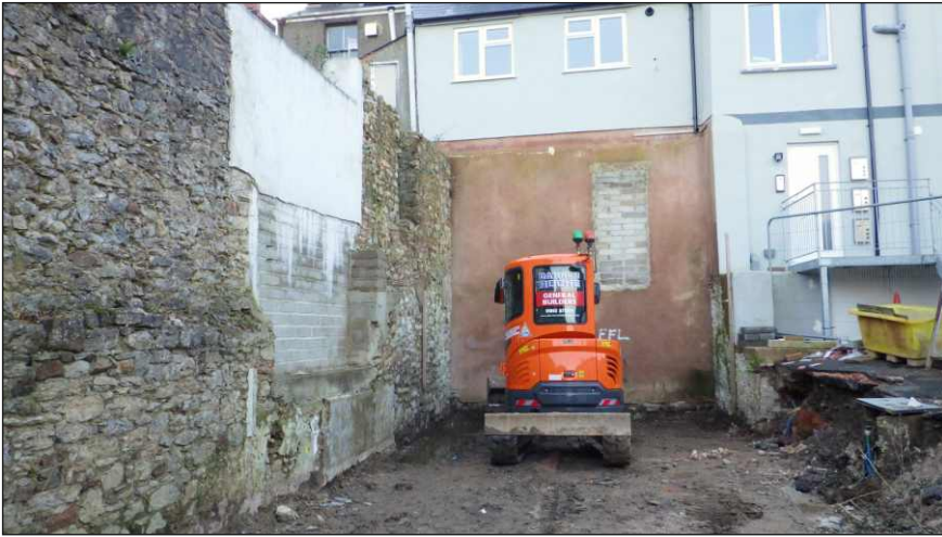
Plate 1: General working view of site looking southeast towards 80 Fore Street
