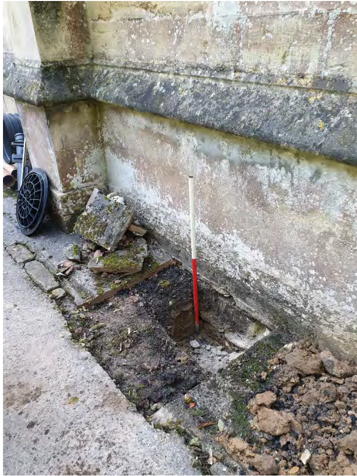
Plate 3. Exposed footings of the 1889 rebuild of the north wall of the nave. View from the north-west
