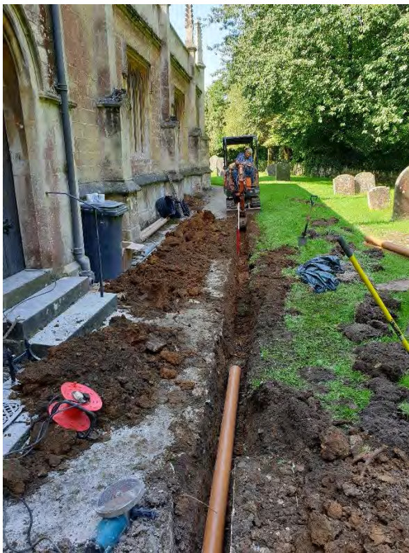
Plate 2. View to the west following excavation of the trench
