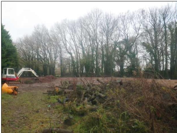
Plate 7: General working view of Area C, Profiles 5 and 6, looking north
